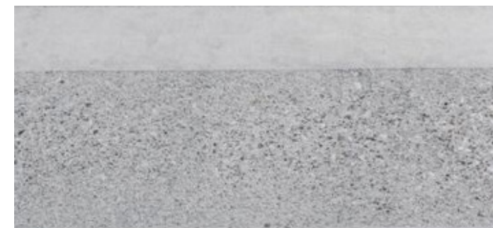
EXAMPLE IMAGE: IN SITU CONCRETE TEXTURE CHANGE (SLIP-RESISTANT)
