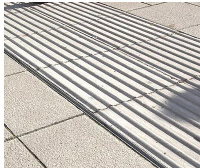
CORDUROY HAZARD PAVING
