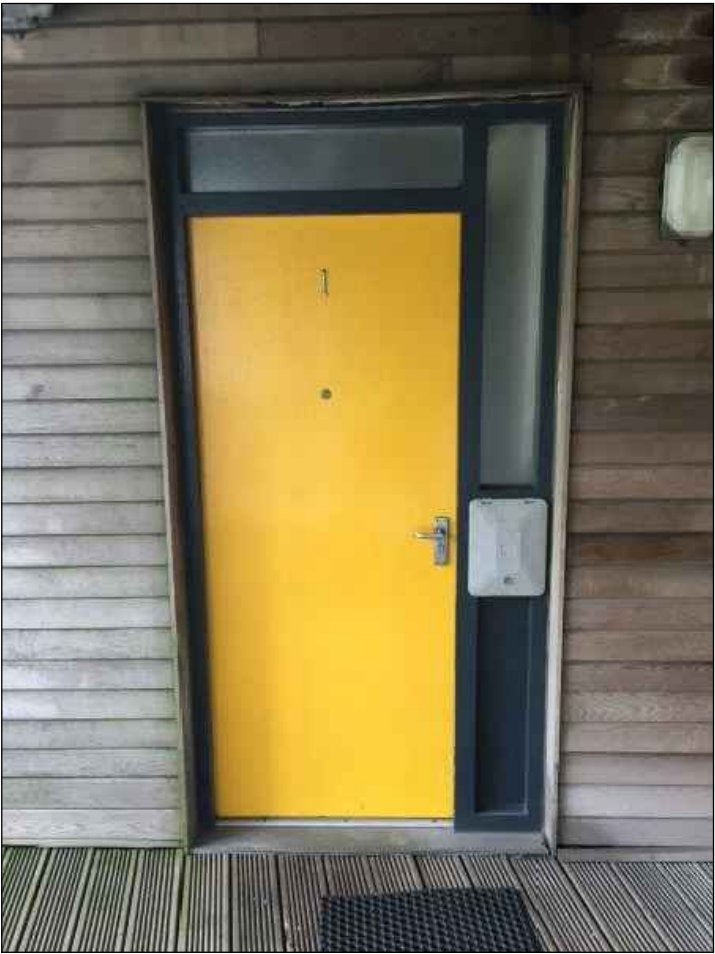
IMAGE OF EXISTING DOOR SET TO BE REPLICATED - APPROX 60 DOOR SETS IN TOTAL
