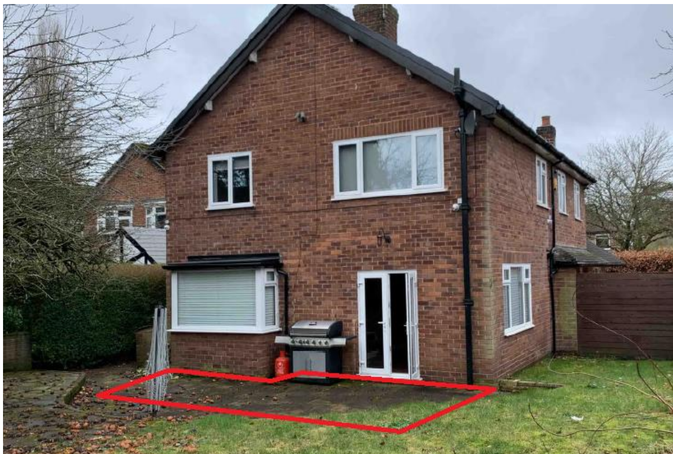
View of east facing elevation where extension is proposed to be erected
