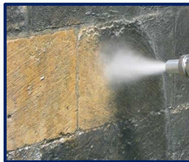
The TORC system being used to remove carbon sulphation from Canterbury Cathedral.
