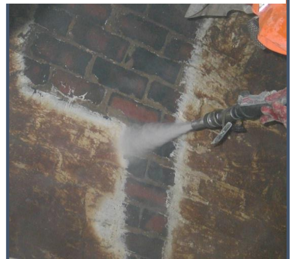
The TORC being used to remove many layers of paint from inside Paddington Station
