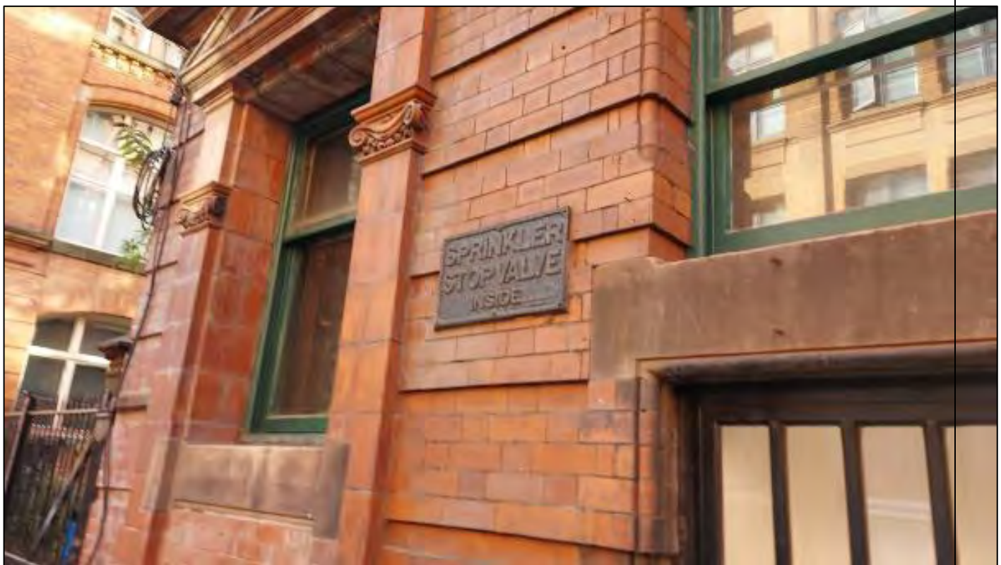
Sprinkler sign retained.
