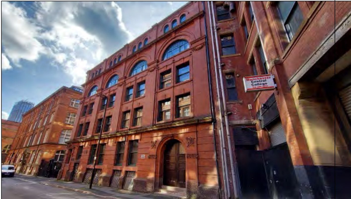
With box sign removed,.
