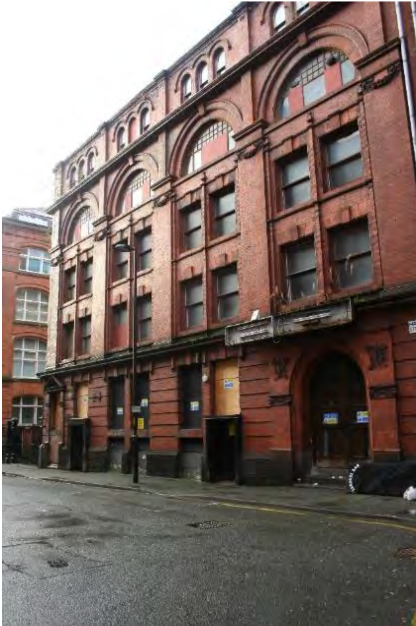
Box sign before works
