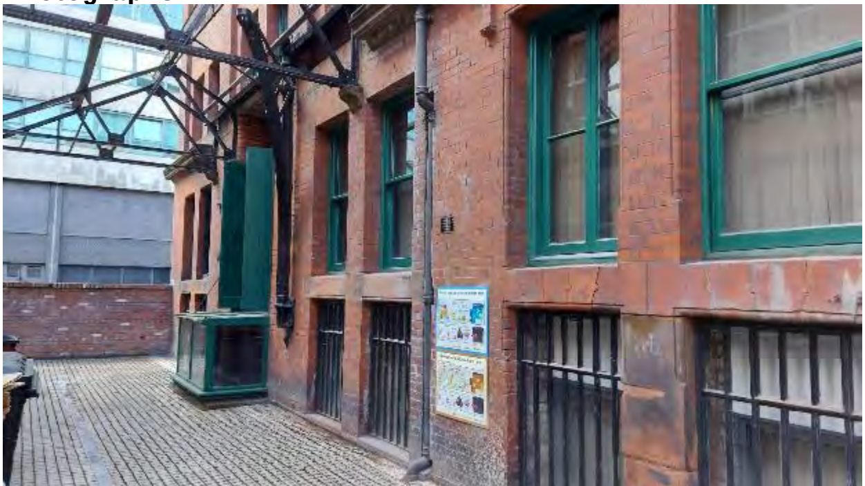
The side elevation loading doors retained in situ and pointed.
