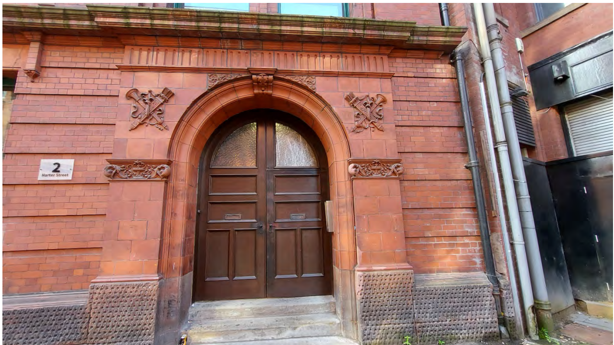
The entrance door after works.
