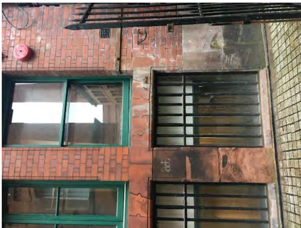
The new windows to the side elevation.
