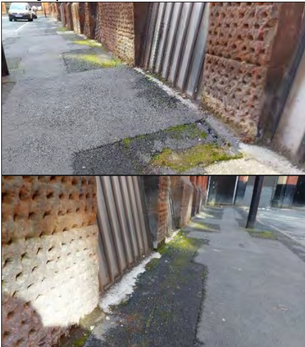
Works to pavement / basement junction.
