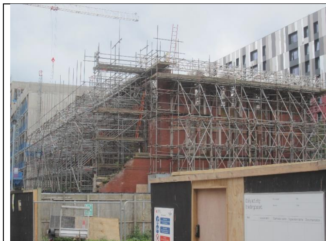
Photo 1: South-eastern and north-eastern elevations
