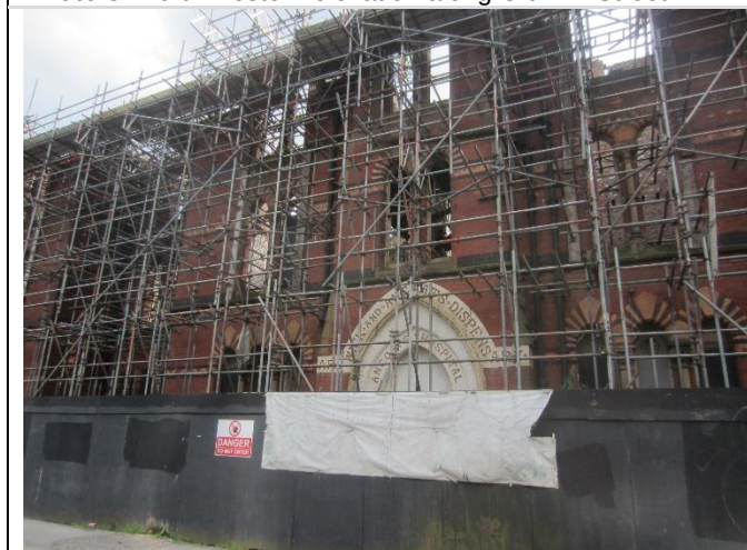
Photo 5: Brick façade of building at north-western elevation
