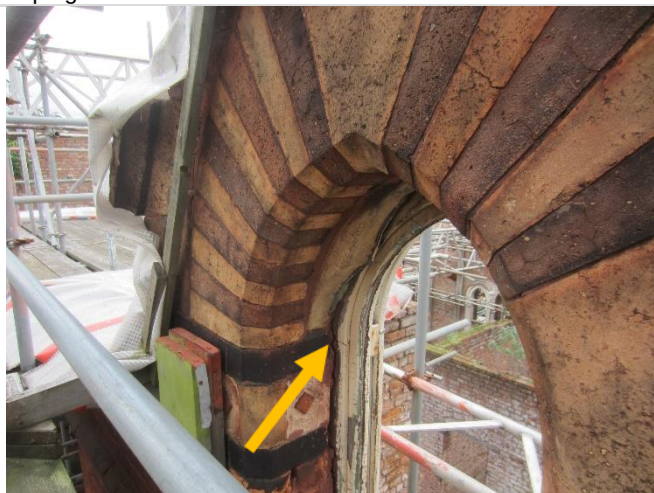
Photo 12: Gaps around the rotten timber window frames were examined with torches and an endoscope to search for bats and evidence of previous use by bats
