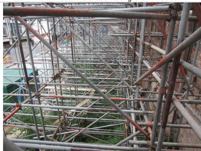
Photo 6: Extent of scaffold supporting the building
