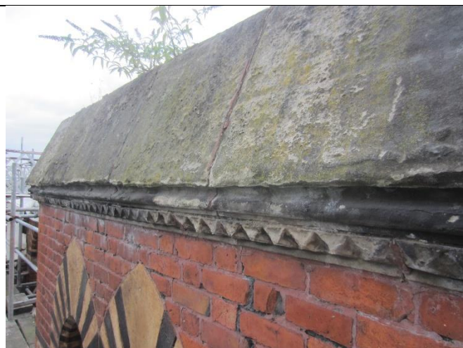
Photo 14: Large and well-mortared coping stones present
