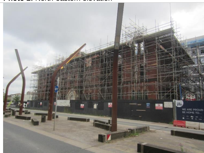
Photo 4: North-western elevation along Old Mill Street
