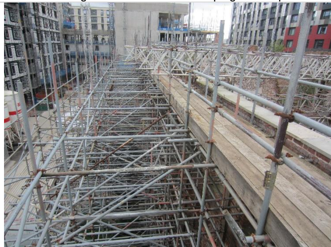
Photo 16: Extent of complex scaffold supporting the building
