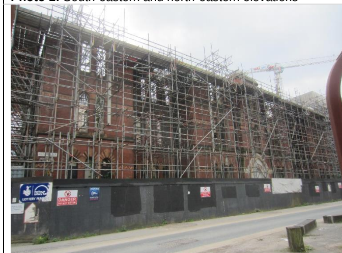
Photo 3: North-western elevation along Old Mill Street
