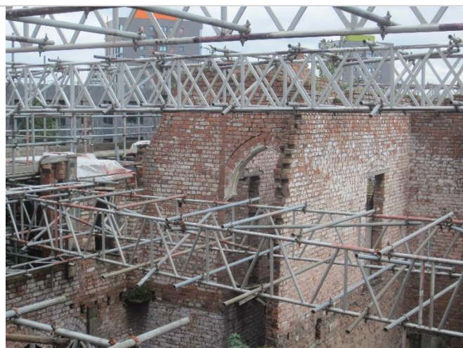
Photo 9: View of exposed brickwork at internal areas
