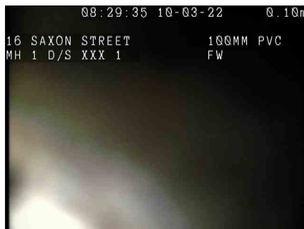
MH 1X_4712a17a-8e59-4a9c-b6b3-05c8fee8da1a_20220310_133 434_199.jpg, 00:00:33, 0.10 m Survey abandoned, SILT
