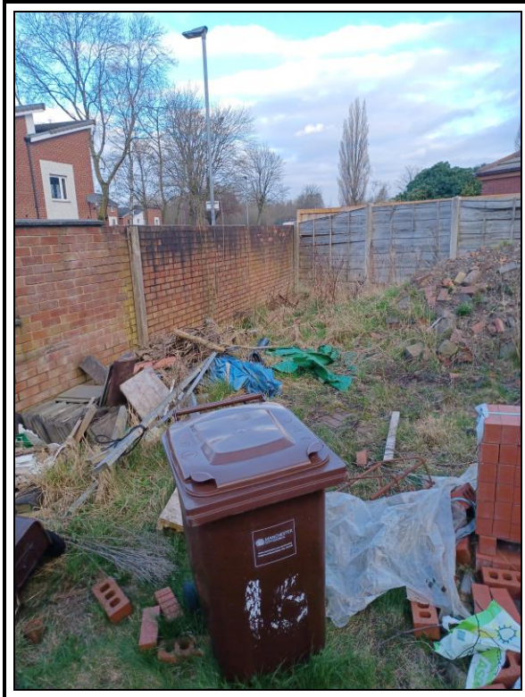
Photo 6, DEBRIS LEVELS ON SITE
