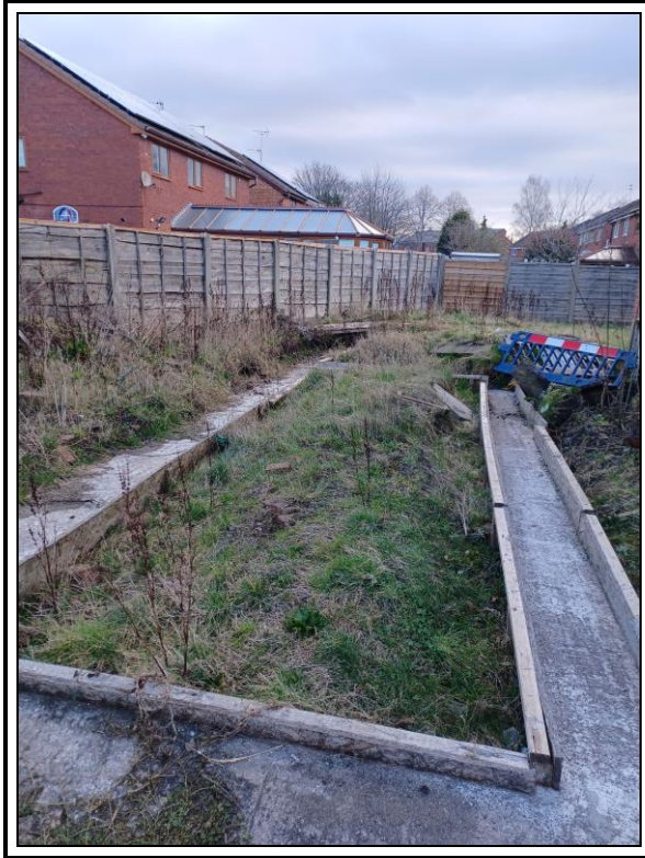
Photo 9, DEBRIS LEVELS ON SITE
