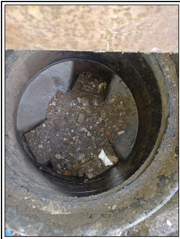
Photo 12, MH2 Silt before removal
