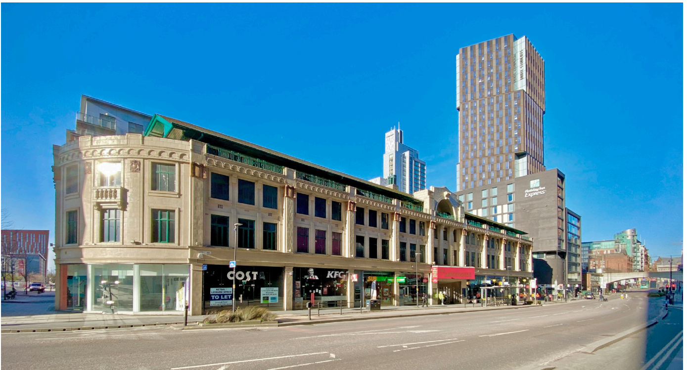
view looking North - 2021 At this point most of the units had been upgraded
