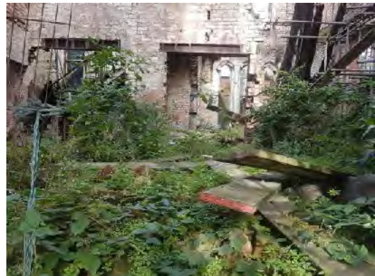
View of ground floor obstructions from the northeast
