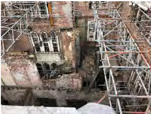
View southwest from the upper northeast perimeter
