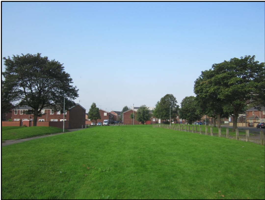
Photograph 4. Existing residential houses on Mayton Street (looking east)
