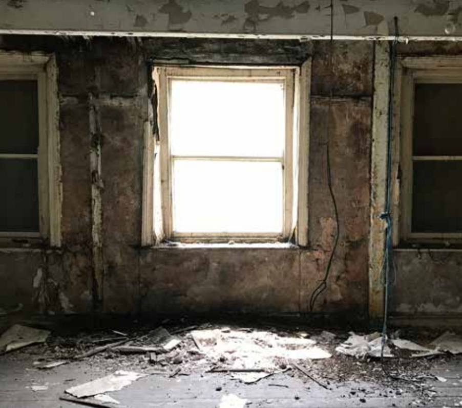
photograph of second floor windows
