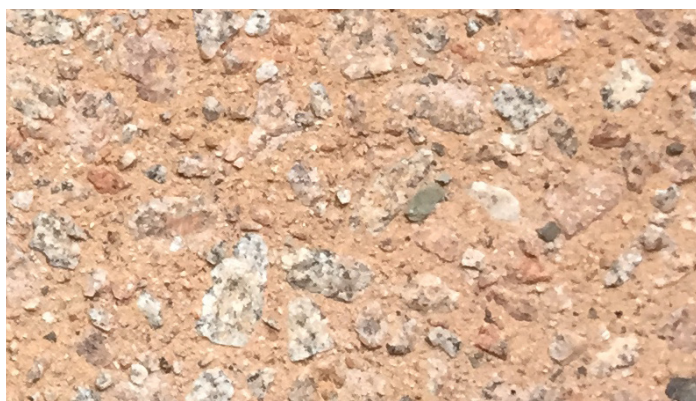
C3 IN SITU CONCRETE
