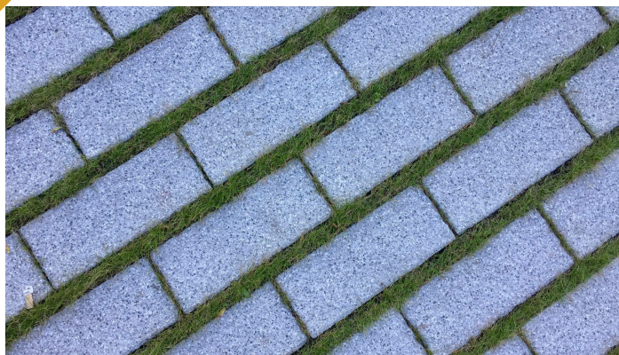
P1 PERMEABLE CONCRETE PAVING -
