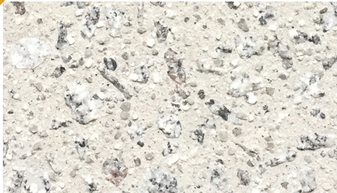
C2 IN SITU CONCRETE
