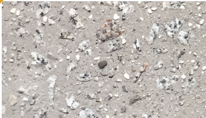
C1 IN SITU CONCRETE
