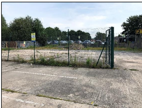
Photograph 1 – Hardstanding within the site.
