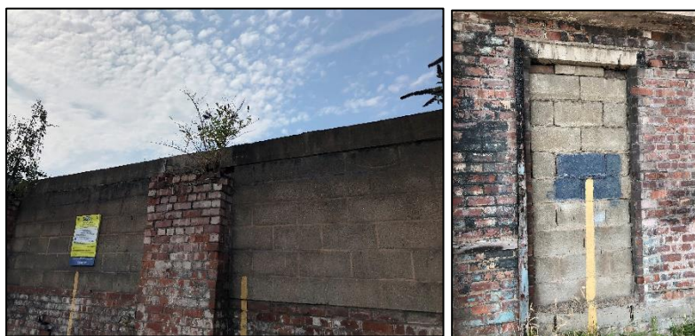
Photograph 6 & 7 – Brick wall on the western boundary of the site
