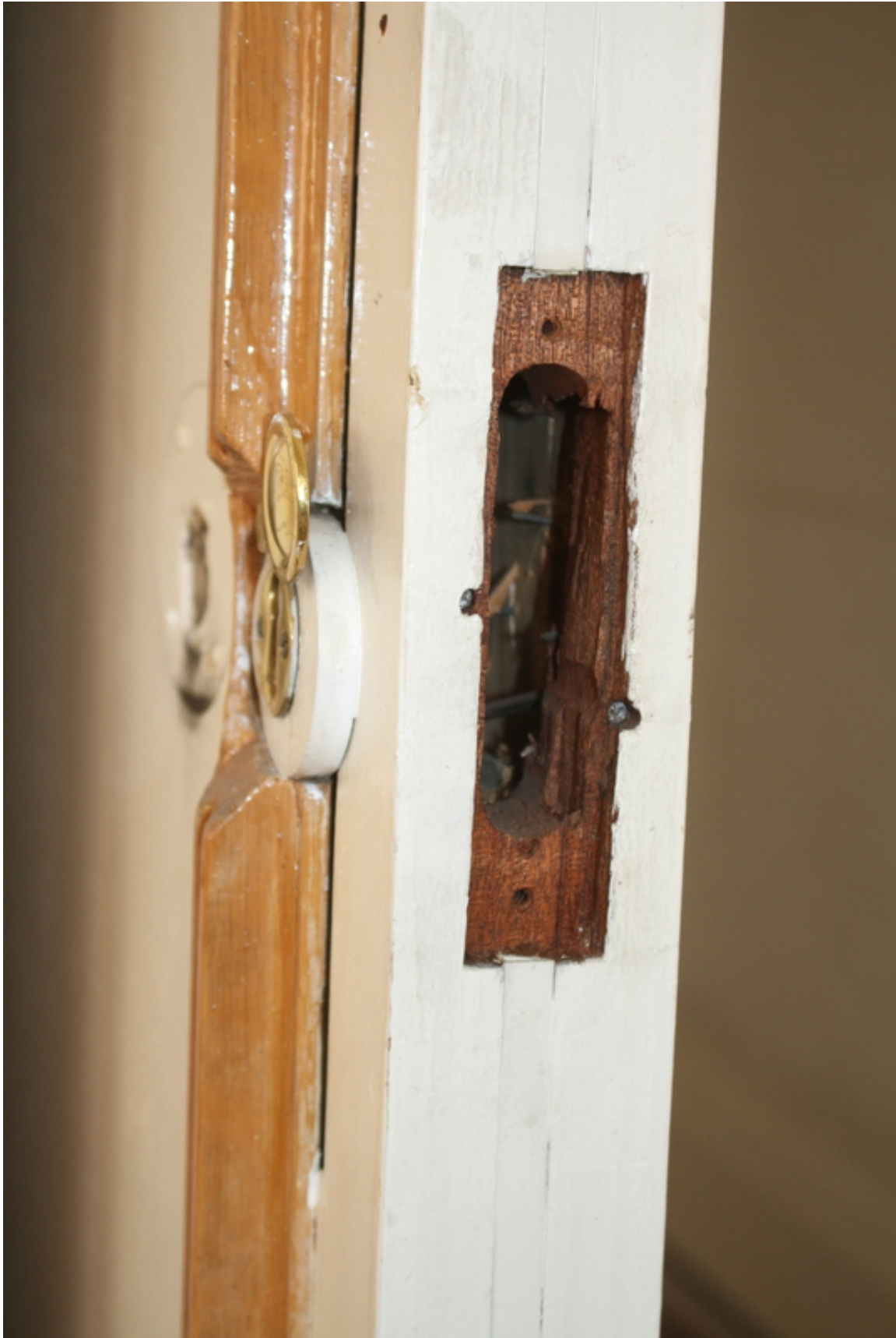
Potential original hardwood elements within some doors
