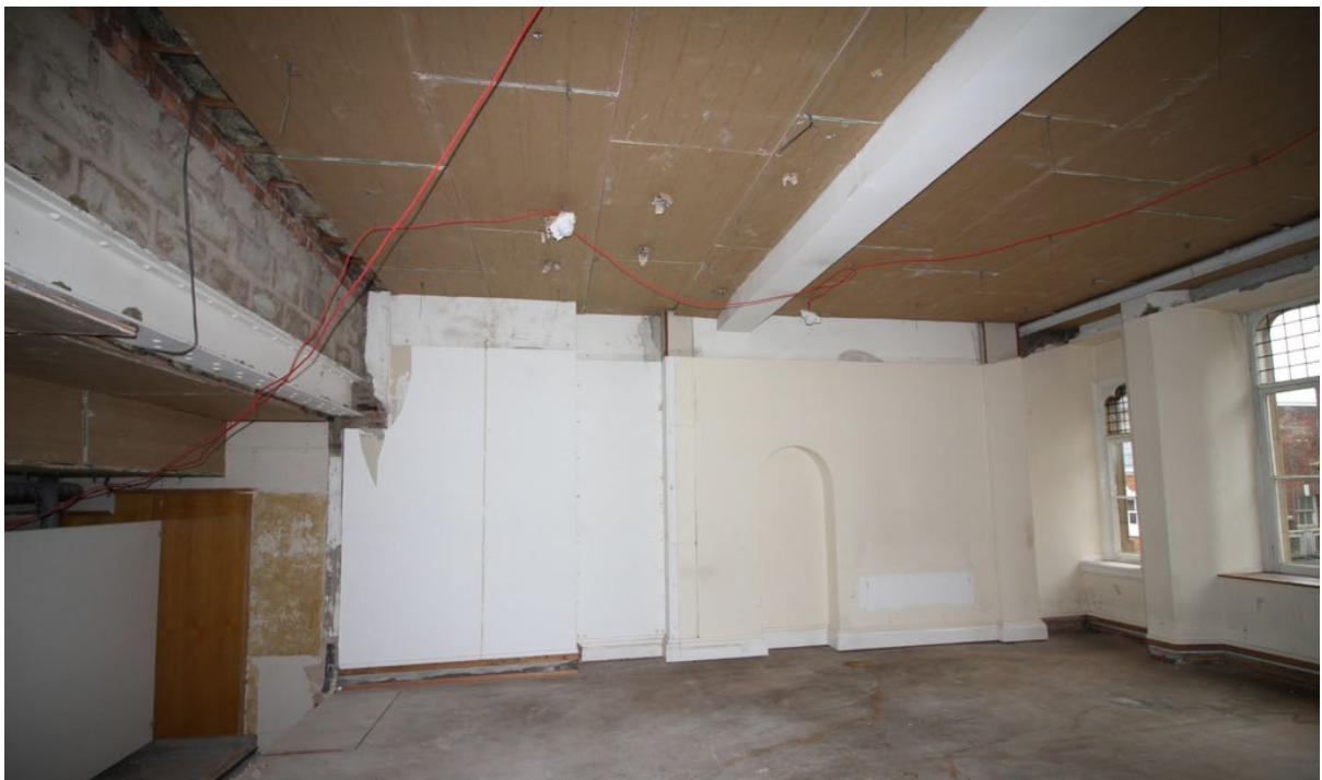
Second floor ceiling in northern room, showing inserted steel beam, and modern plaster overlying earlier wall plaster
