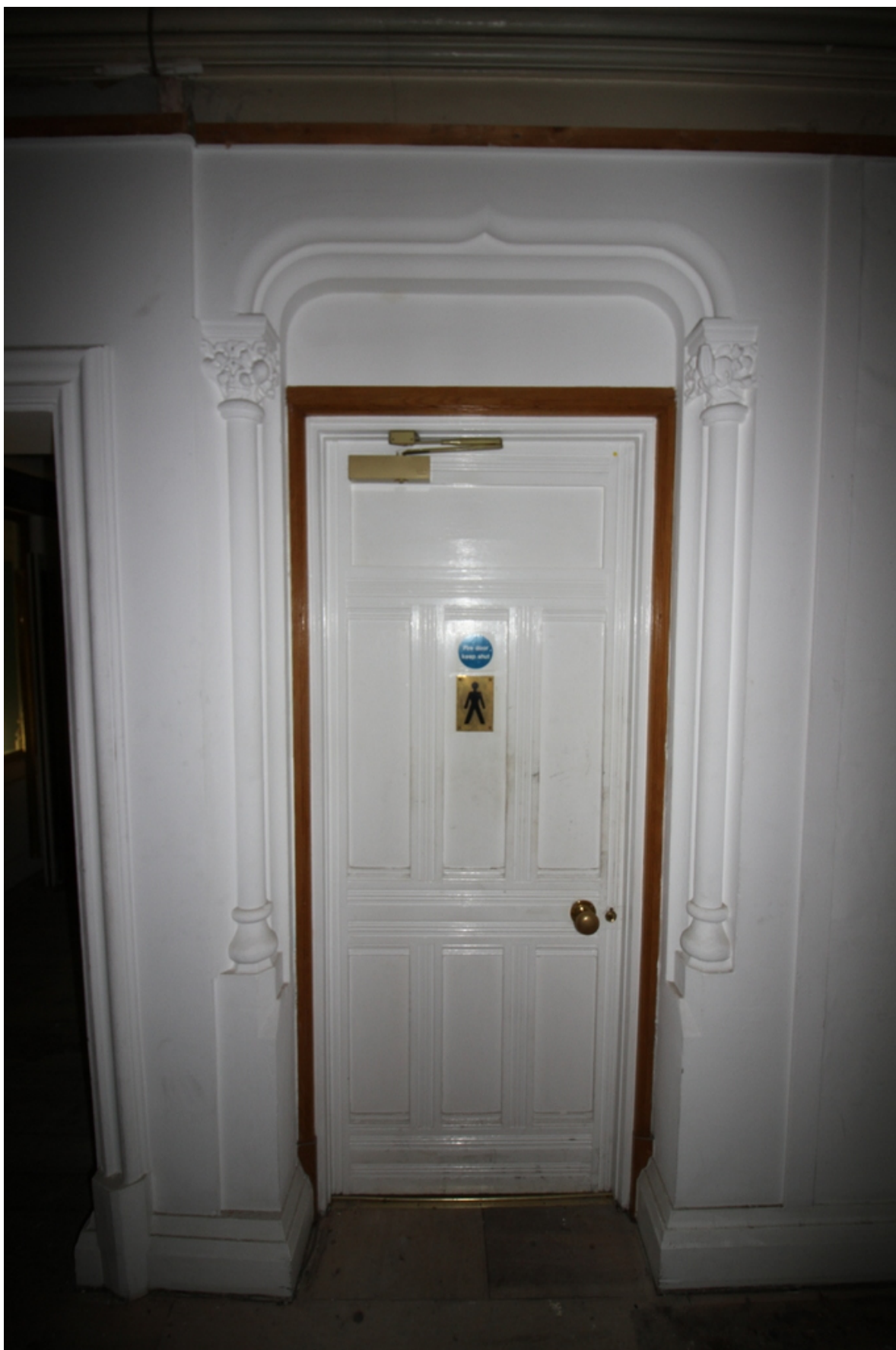
Decorative moulding surround to extant doorway 62 King Street second floor
