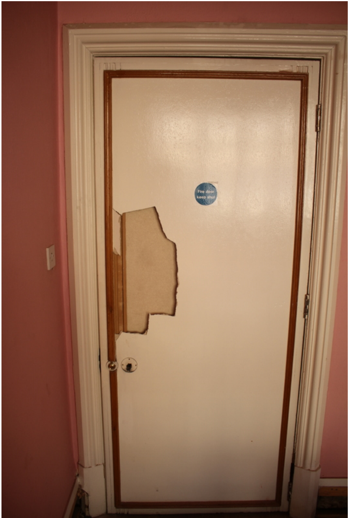
But panels replaced with fireproofing
