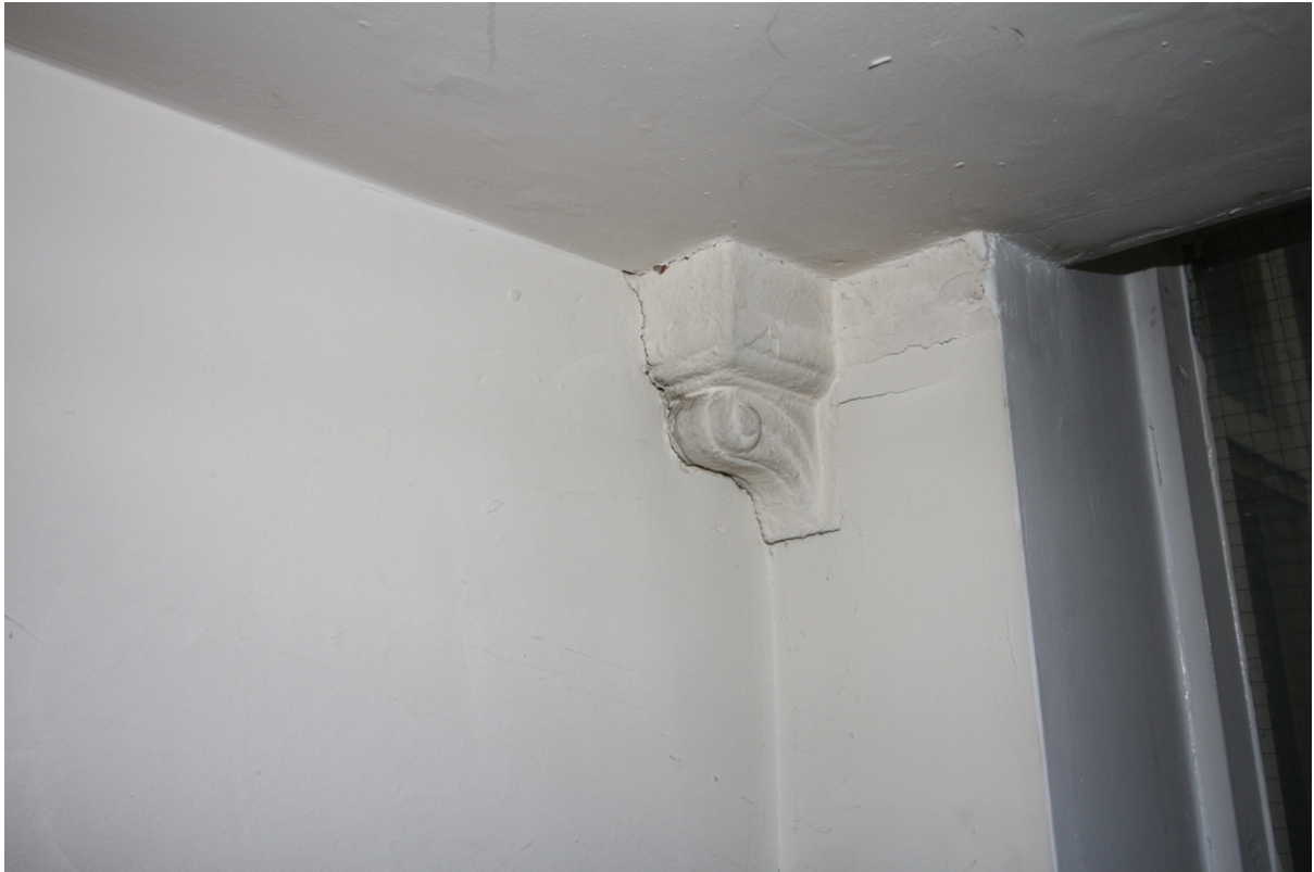
Corbel within stairwell of 58 King Street, first floor
