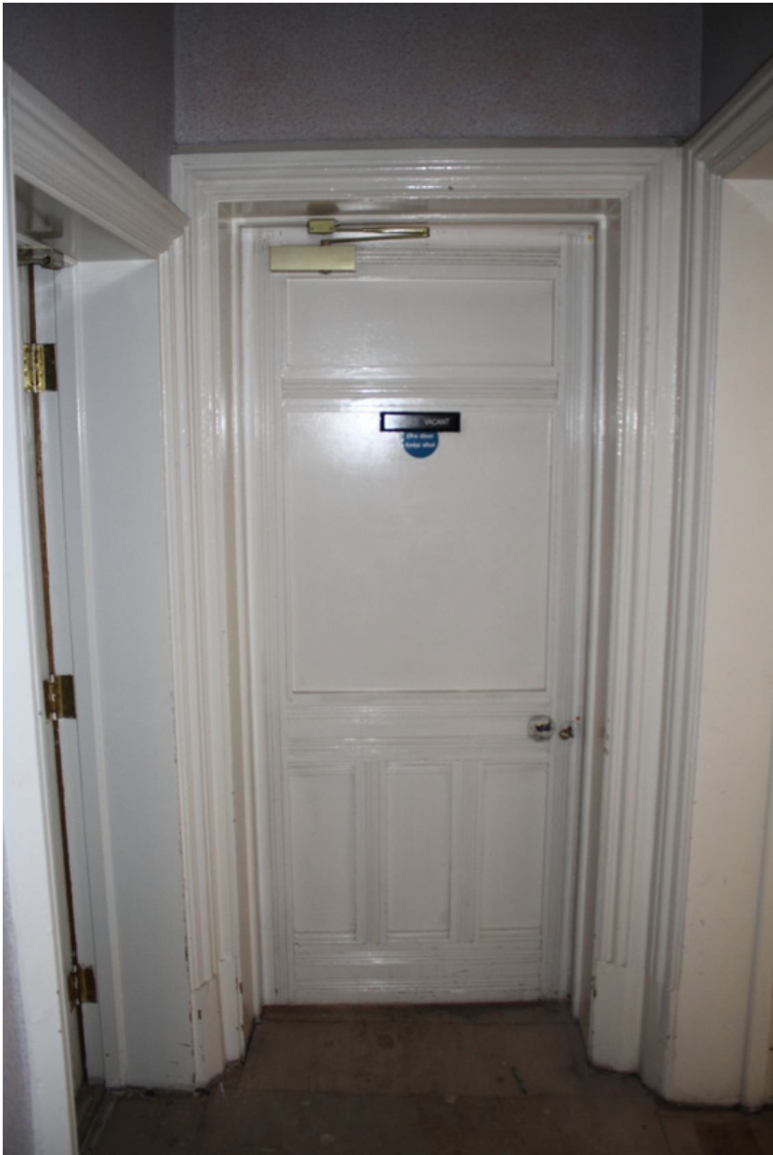
Moulded architrave and panelled doors
