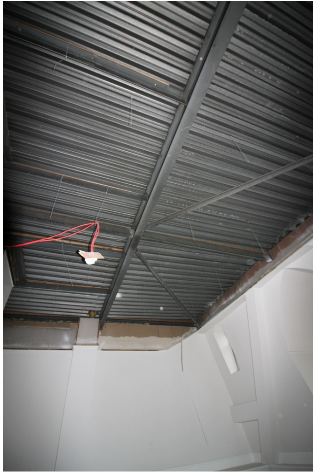
Late-20 th century roof structure within northern part of listed building, 3 rd floor
