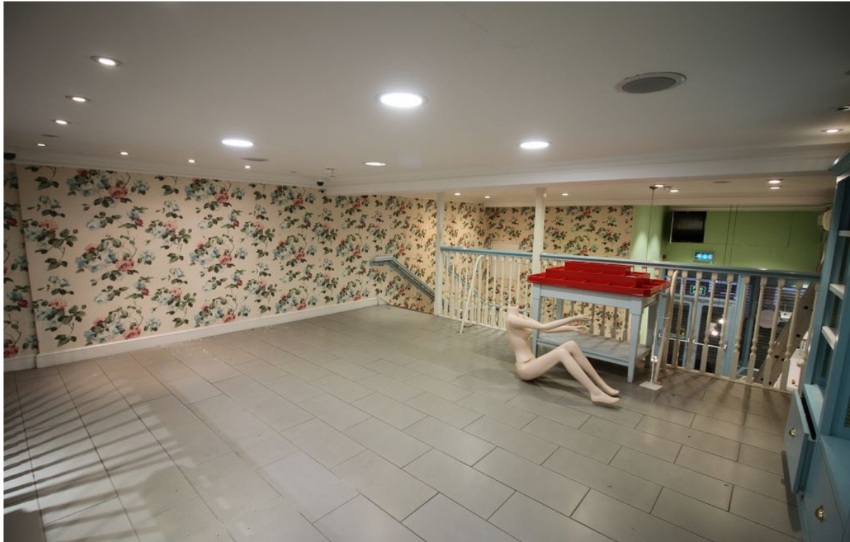
Late suspended ceiling, wall finishes and inserted mezzanine floor within ground floor shop
