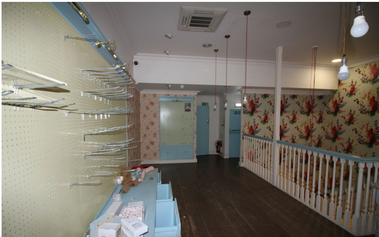
Late suspended ceiling, wall finishes and inserted partition walls within first floor level of shop
