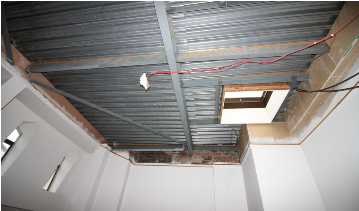
Late-20 th century roof structure within southern part of listed building, 3 rd floor. Modern wall finished can be seen above the line of the suspended ceiling
