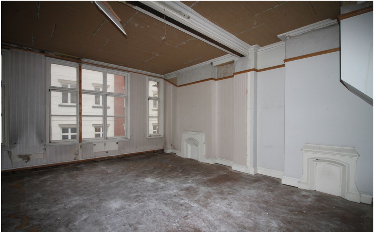
First floor ceiling in southern room, and retaining possibly original wall plaster
