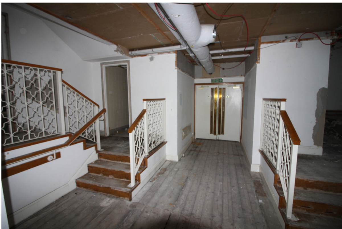
Second floor ceiling within central inserted corridor with late stairs
