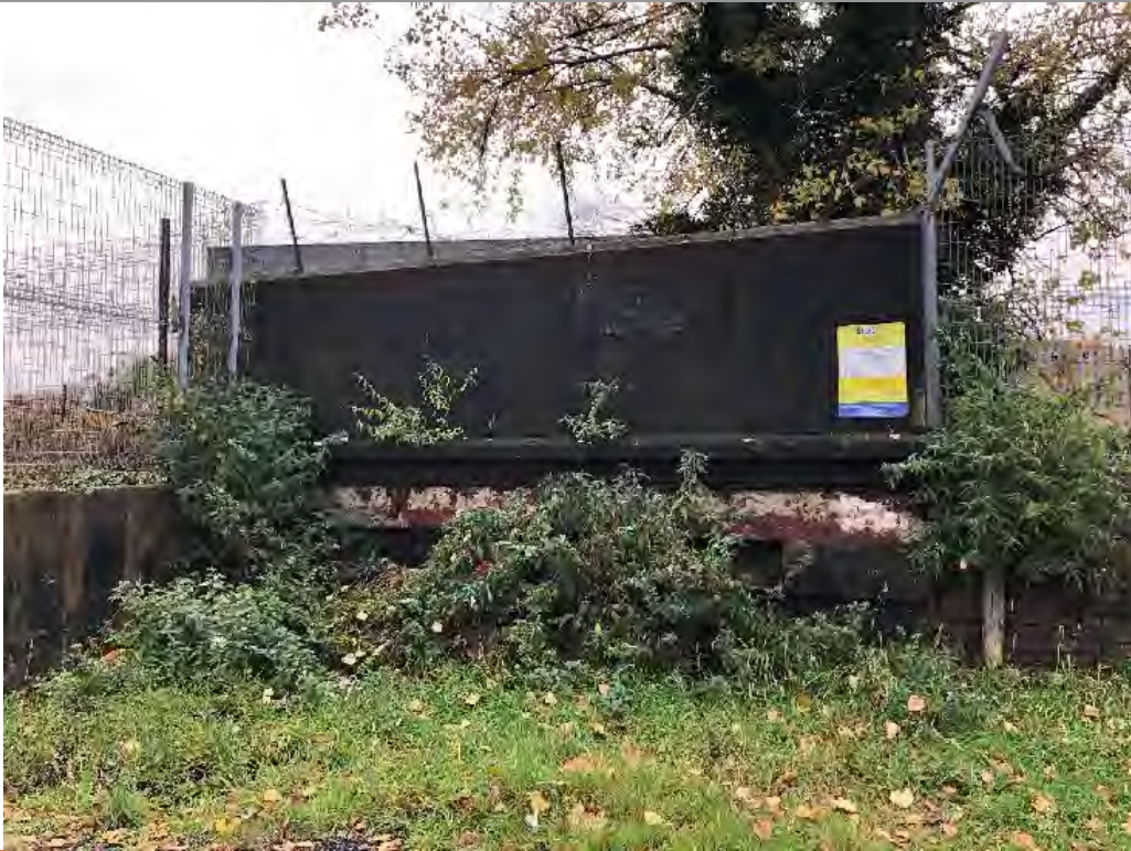
PLATE 1 PARCEL B BRIDGE STRUCTURE UNDER JERSEY STREET LEADING TO PARCEL C
