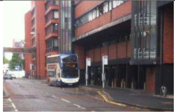
Photograph 6.10 Booth Street West Westbound bus stop
