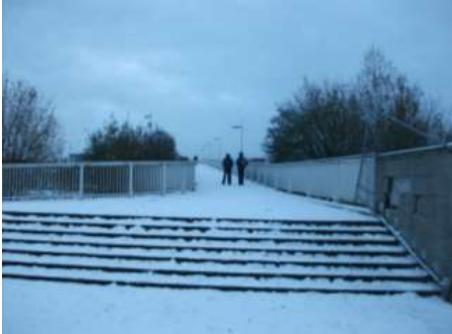
Photograph 6.3 Princess Road Footbridge
