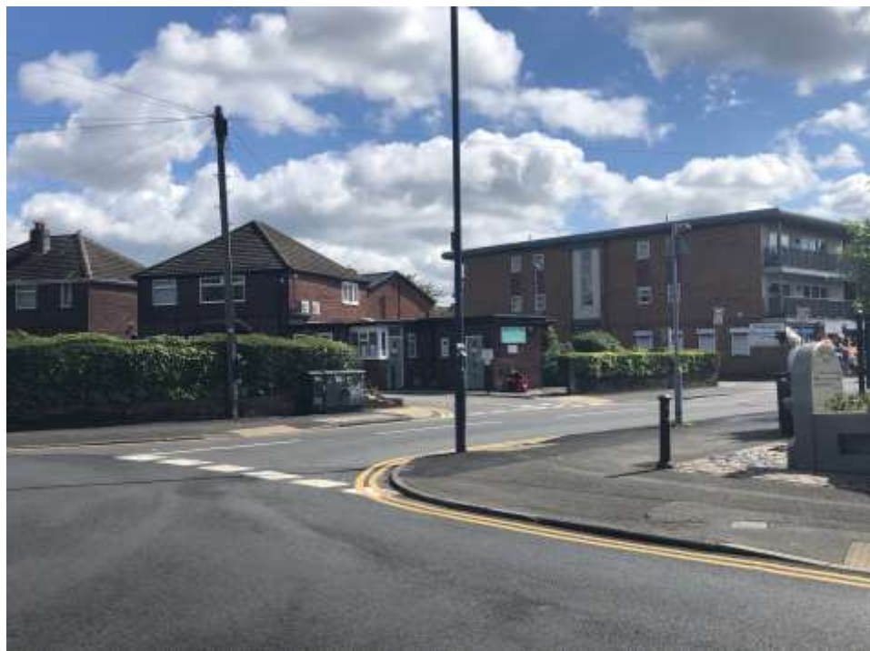
Below: Photo looking at the site from Old Moat Lane from across the roundabout
