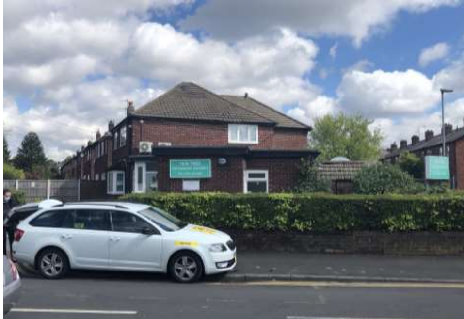
Above: Photo of the south elevation
