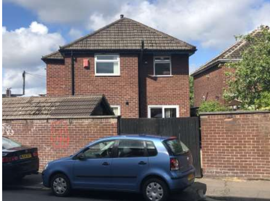
Above: Photo of the east elevation showing existing gated access to the rear of the property off Hill Street
