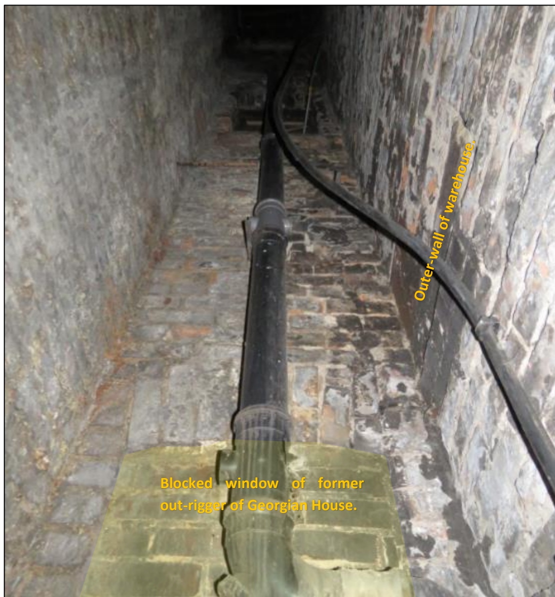
Figure 59. View of the internalised shaft created by the enclosure of the much-altered remnant of the out-rigger of the former Georgian House.
