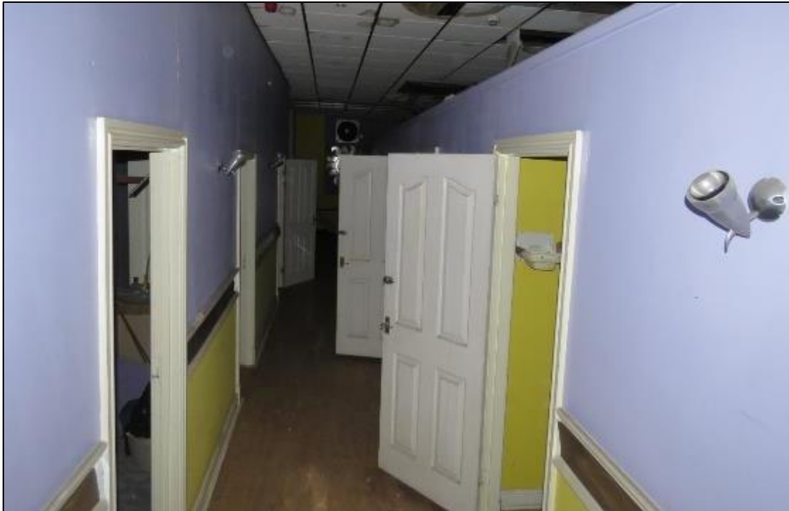
Figure 46. The interior of the first-floor of the warehouse, as accessed from the landing (March 2019).
