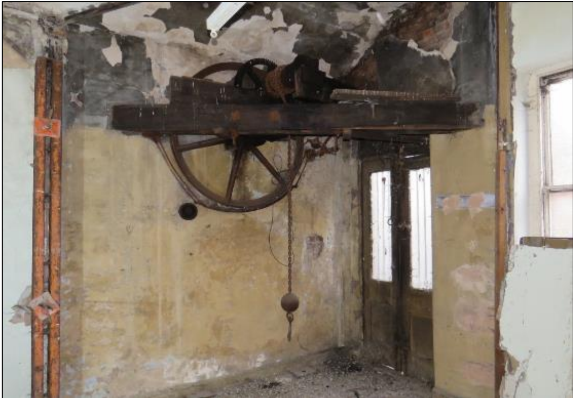
Figure 55. The surviving warehouse hoist and the bringing-in doors facing Back Piccadilly (March 2019). The internal nature of the hoist emphasises that this is a late-C19th warehouse as it post-dates the local by-law which required loading to be off-street.
