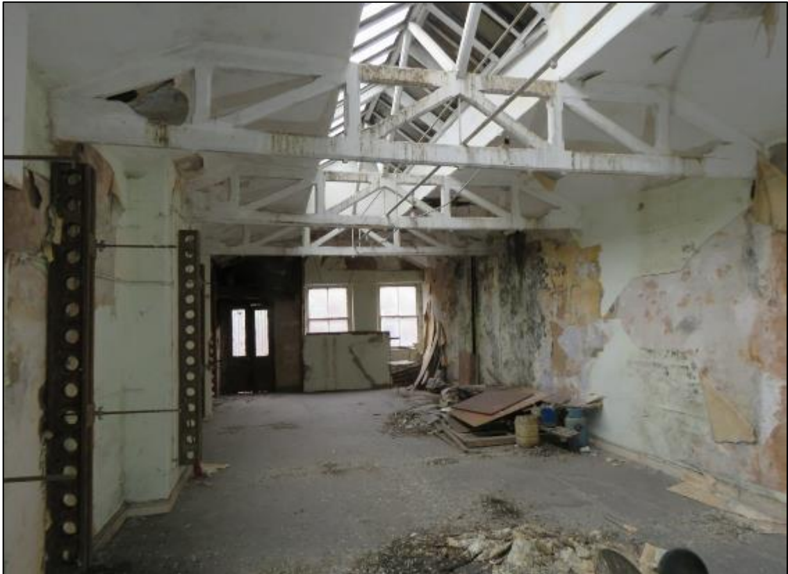
Figure 53. View into the second-floor of the warehouse (March 2019), looking towards Back Piccadilly. The roof trusses are supported from the adjoining wall and support the roof-light. The wall retains the original -late-C19th plaster but is other-wise a simple storage space.
