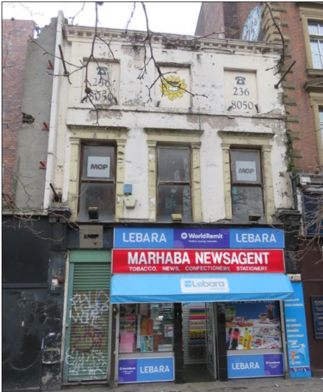
Figure 56. The altered Piccadilly elevation (March 2019). This is the key, character defining elevation but is dominated by the modern shop-unit (which overlays the c1909 Midland Railway Company changes). The first-floor windows are modern replacements. The left-hand side reveals the remnant of the rebuilt premises at 43-45 Piccadilly which abuts the surviving dentilled cornice.
