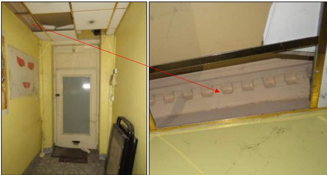
Figure 40a. View looking south toward the entrance with surviving Georgian plaster cornice.
