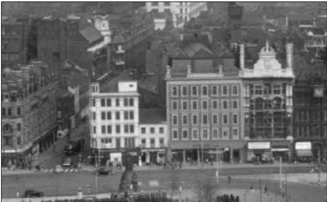
Figure 57 The Piccadilly frontage c1960, showing the juxtaposition of the surviving Georgian premises with its neighbours.
