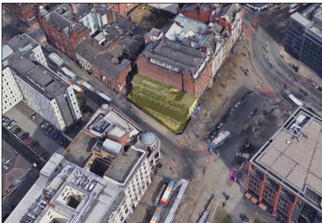
Figure 2. Aerial view of the site looking east, showing the three distinct components: cleared site, former town-house and warehouse.
