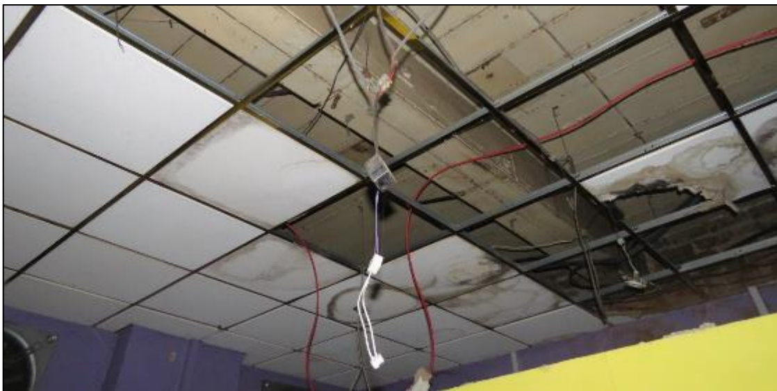
Figure 47. Inserted ceiling of the first-floor warehouse with the under-side of the floor-boards on the second floor partially exposed (March 2019). The main beams are supported in shoes from the flanking brick-wall as on the lower floor levels.
