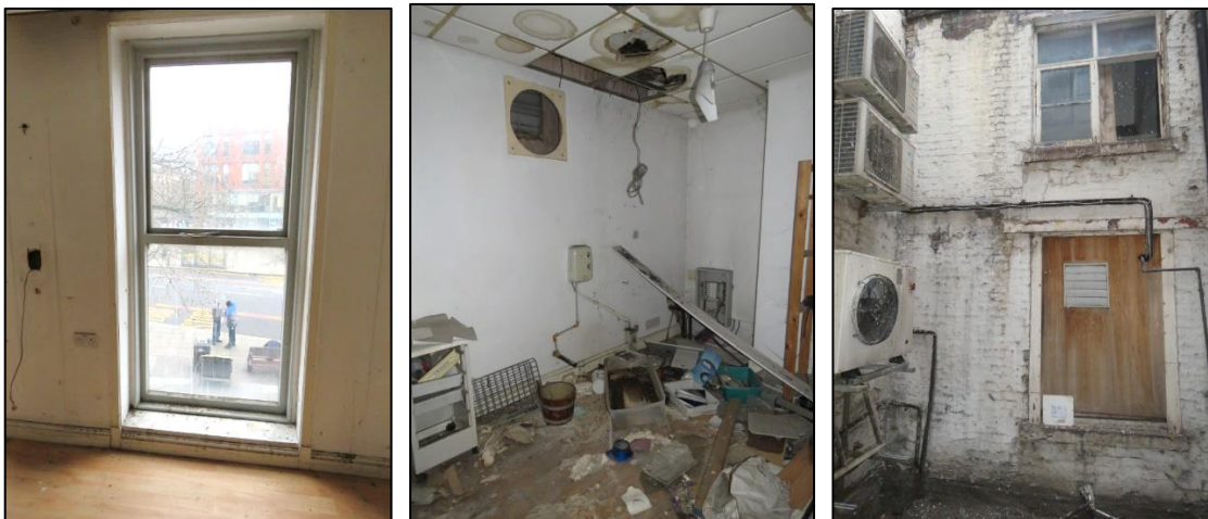
Figure 45. The front (LHS) and rear windows of the much-altered first-floor of the former dwelling.
