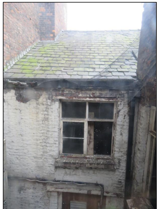
Figure 52. Rear view of the second-floor from the warehouse (March 2019)
