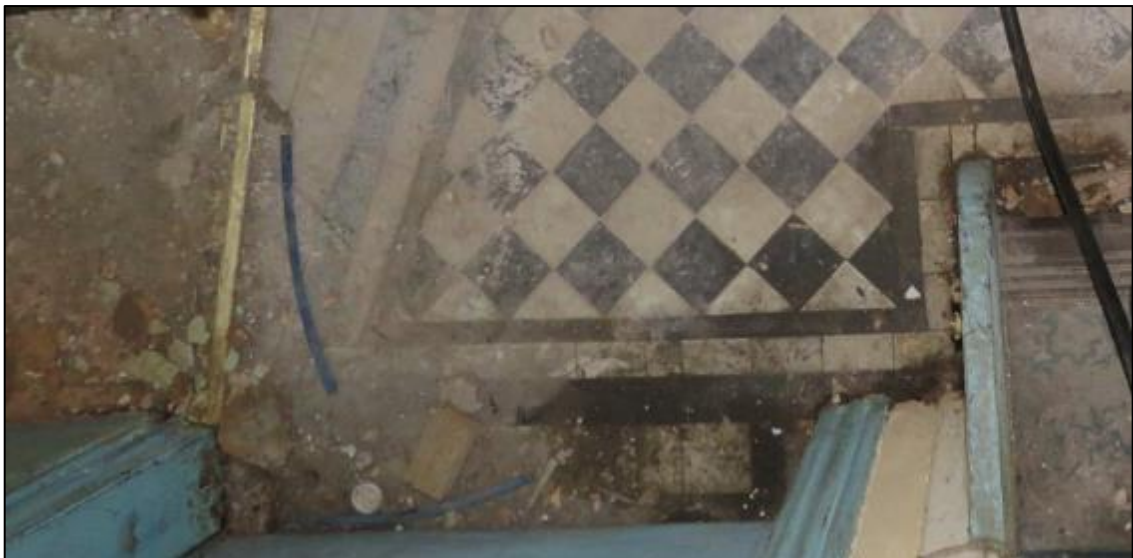
Figure 36. Late-C19th tiled-floor at the base of the stairs (03.06.19).
