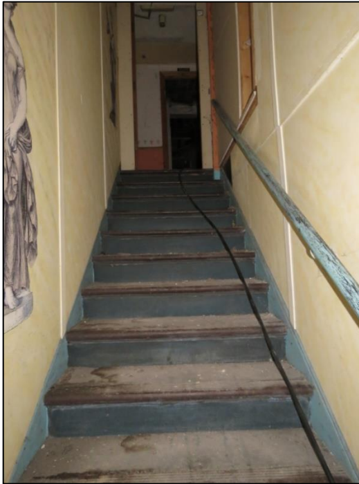
Figure 34. Stairs to the basement (03.2019).
