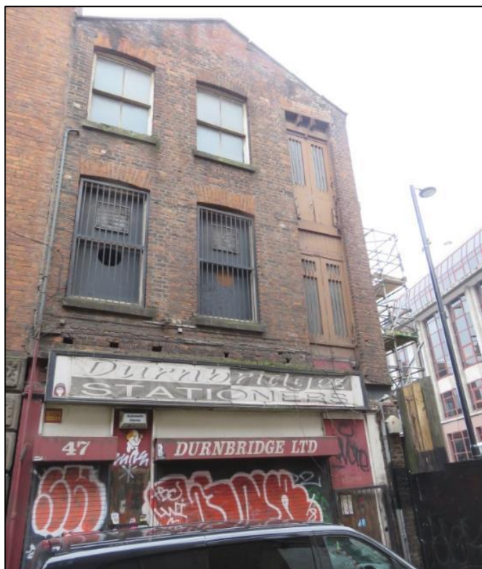
Figure 62 The Back Piccadilly Street elevation (March 2019) showing the repairs and alterations.
