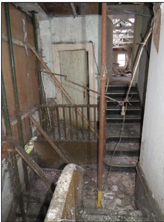
Figure 51. The landing connecting into warehouse.
