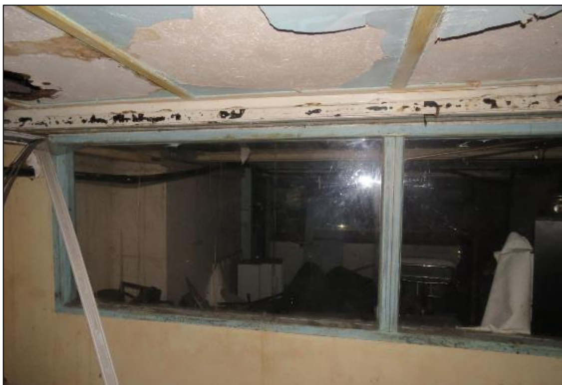
Figure 33. View of the basement modern partitions and plaster ceiling (March 2019).
