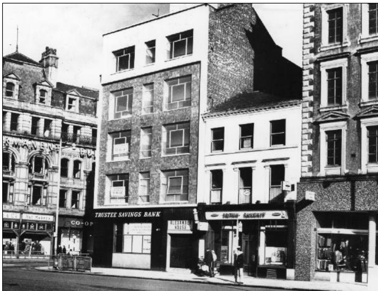
Figure 31. View of the remodelled premises (1967) at 43-45 Piccadilly and early-C20th shopfront at 47 Piccadilly which retained separate access to the upper-floors and rear warehouse.
