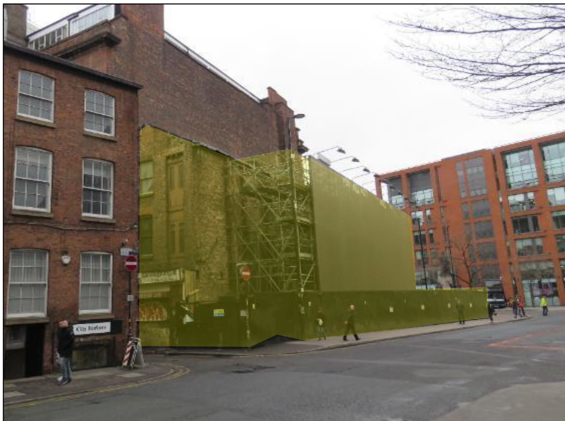
Figure 3. View of the extant site, looking south along Lever Street (March 2019)
