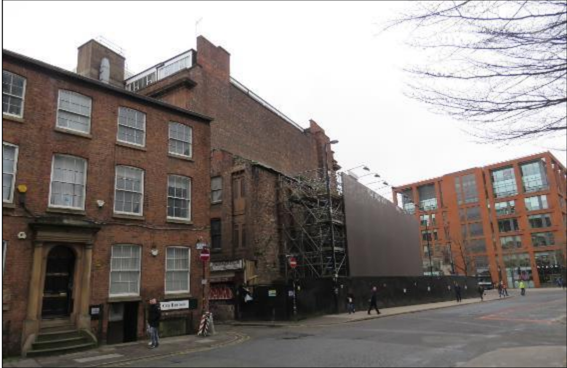
Figure 6. View of 43-47 Piccadilly from Lever Street emphasising the void in the townscape.
