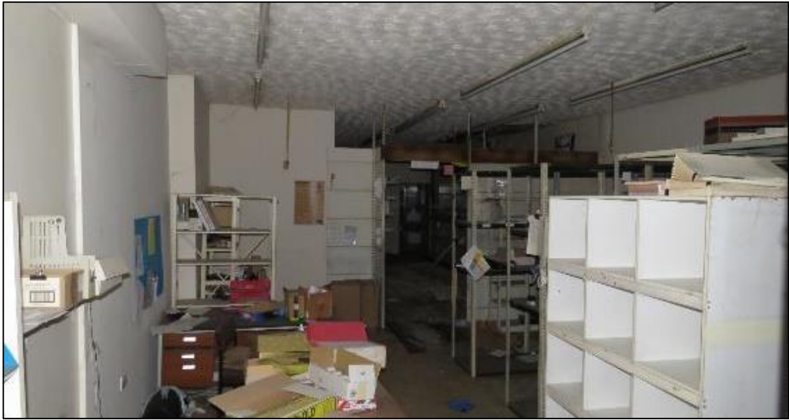
Figure 42 Ground-floor warehouse interior, looking toward Back Piccadilly (March 2019).
