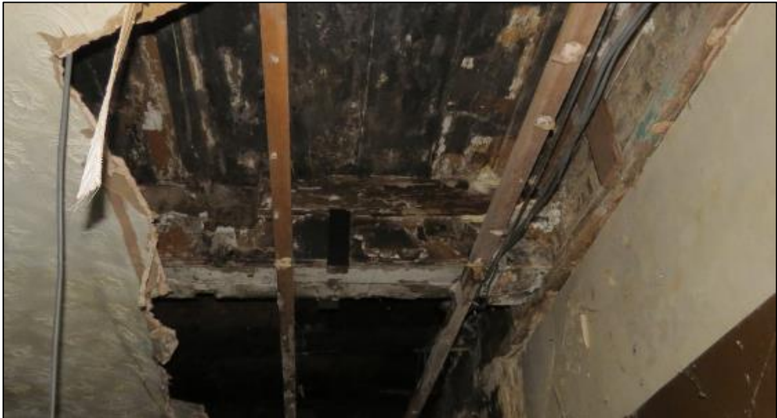
Figure 43 Ground-floor warehouse ceiling showing the under-side of the floor-boards to the first floor and the cast-iron wall-bracket supporting the beam from the adjacent wall of 49 Piccadilly (March 2019).
