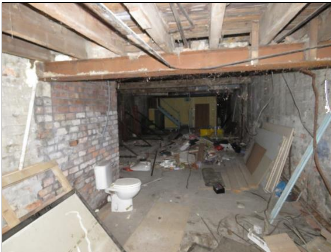
Figure 32. View looking into the warehouse basement (March 2019) from the former dwelling's basement. The left-hand side of the view has the rebuilt section of the former outrigger. The steel-beam is the approximate line of the light-well.
