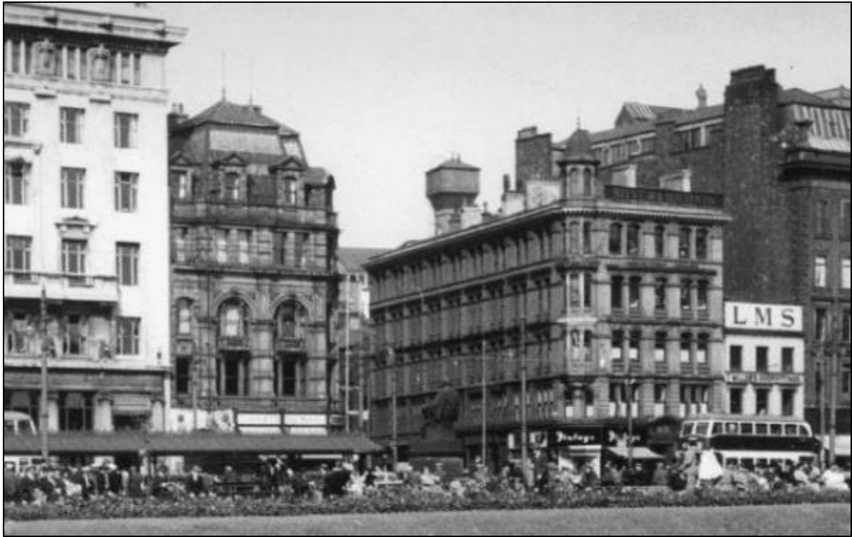
Figure 29. View looking toward 43-47 Piccadilly from the gardens in 1949 showing the dominance of the now demolished premises over the altered Georgian dwelling.
