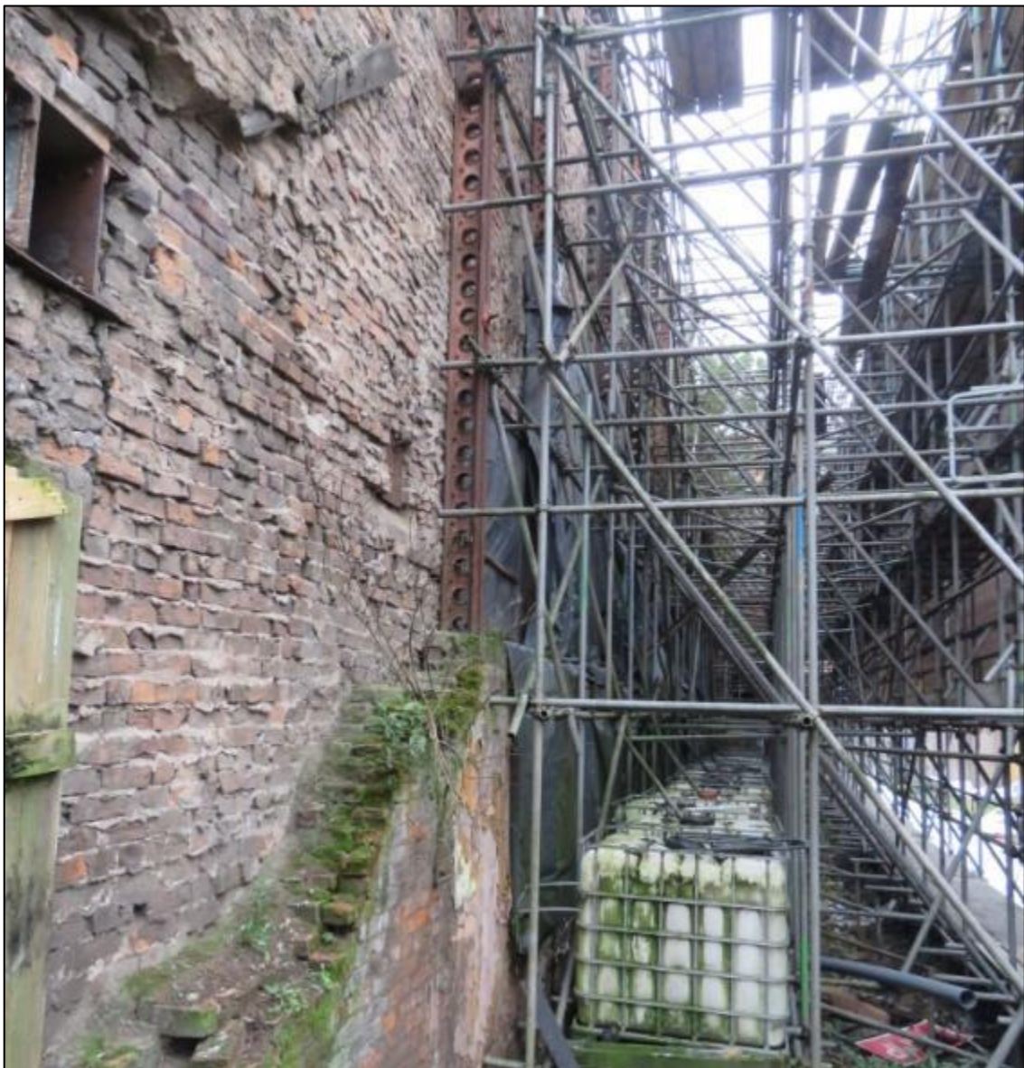
Figure 58. The flank wall to the warehouse component at 47 Piccadilly and the remnant of the load-bearing wall of 43-47 Piccadilly (March 2019). The steel shoring-anchors/braces are connected internally (see below).
