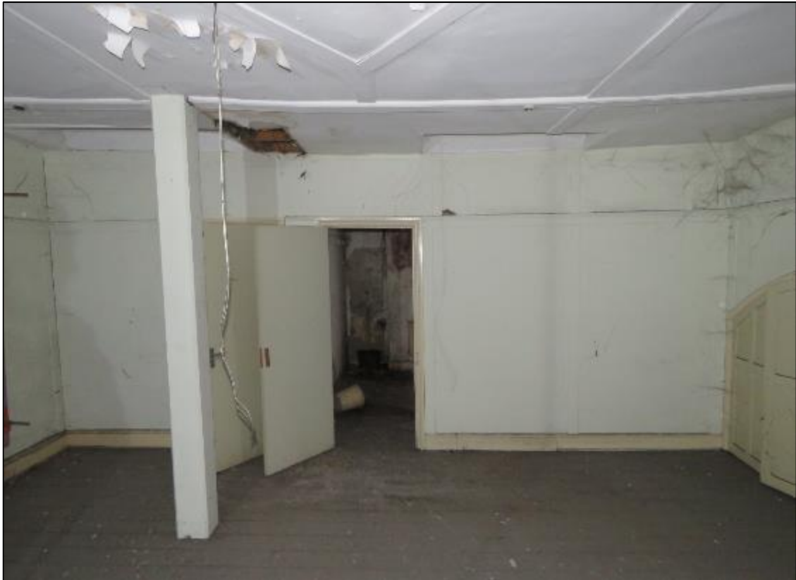
Figure 50. View looking into the rear second-floor room showing the early-C20th fabric and the removed internal walls which now create a main space with an internal access to a rear office (facing into the lightwell). The left hand door accessed the corridor and landing and then directly into the rear warehouse.
