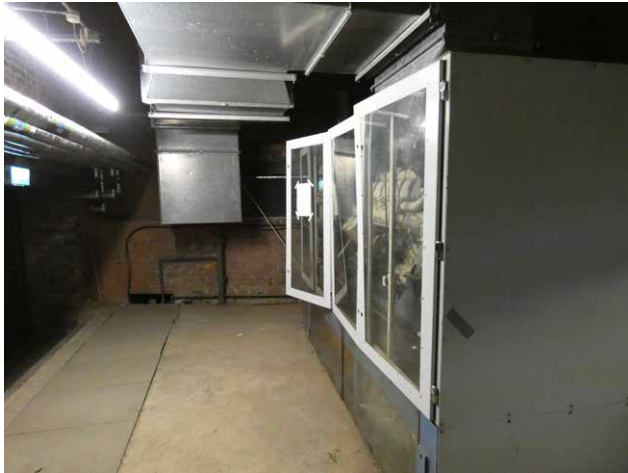
3.26 1830 Viaduct, Arch 2B (Install)
