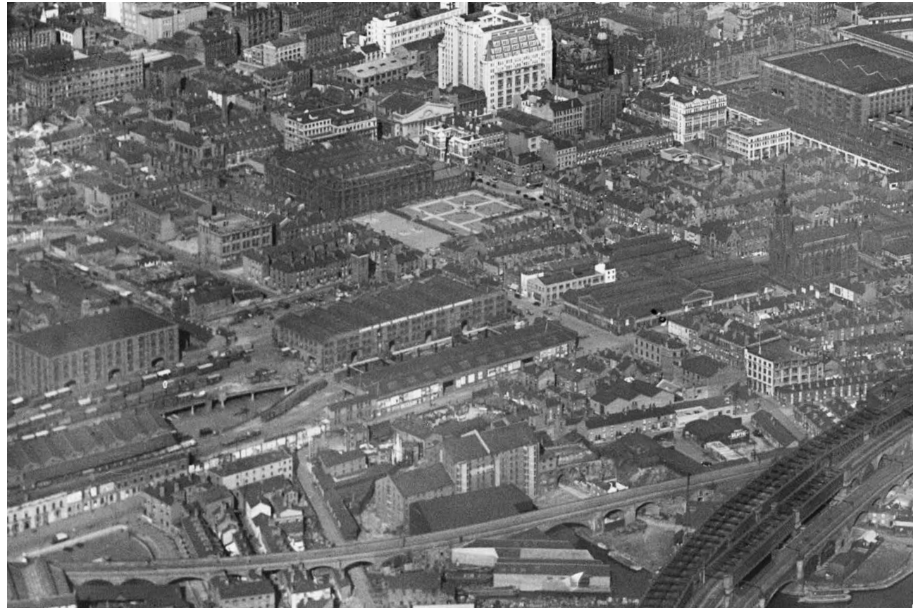
2.5 The City Centre from the South-West, 1934 with Liverpool Road Station on the left (Britain From Above, EPW045993).
