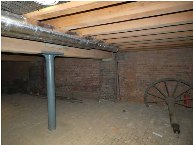
3.24 1830 Warehouse, LG02 looking south (Insall)
