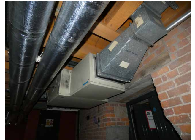
3.21 1830 Warehouse, P01, pipes and plant fixed to modern structure (Insall)
