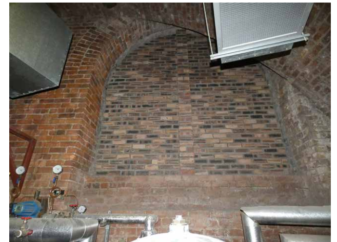
3.31 1830 Viaduct, Arch 3A, north wall (Install)
