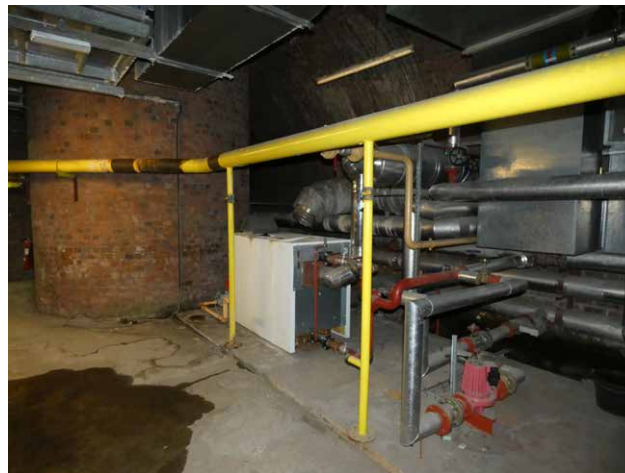
3.30 1830 Viaduct, Arch 3A (Install)
