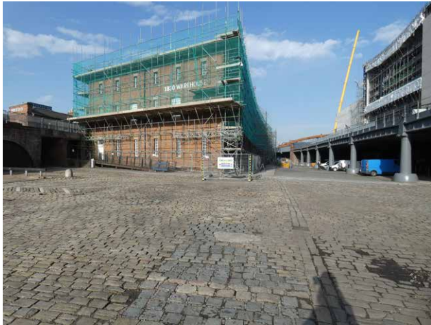
3.12 East elevation of the 1830 Warehouse (Insall)
