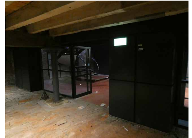
3.18 1830 Warehouse, Stair core LG01 (Insall)
