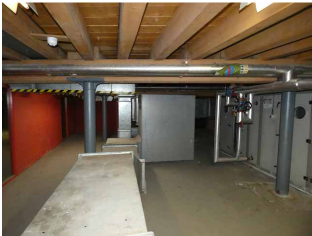
3.19 1830 Warehouse, P01 looking west (Insall)
