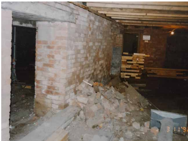
2.14 Internal works to Bay 2, Level 1 (SIM Archive 2015-2002).
