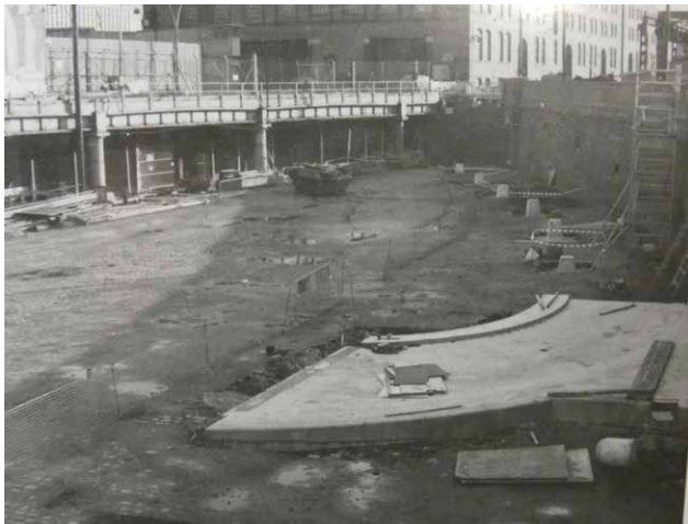
2.18 Construction of the car ramp (SIM Archive YA 2007.41).
