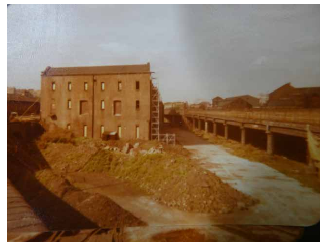
2.8 1830 Warehouse, c.1979 (SIM Archive 2015-2002).
