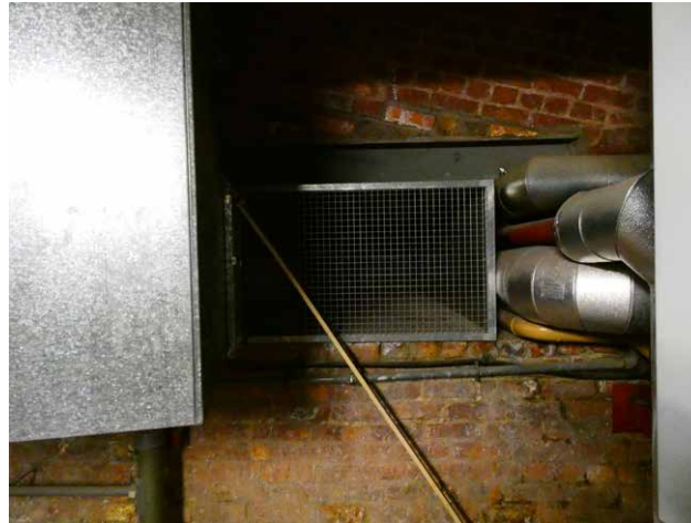
3.27 1830 Viaduct, Arch 2B (Install)
