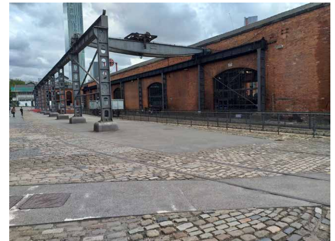
3.6 The Power Hall and Gantry from the Upper Yard (Studio Downie)
