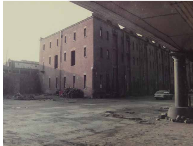
2.10 East and north elevations of the 1830 Warehouse, c.1990 (SIM Archive 2015-2002).
