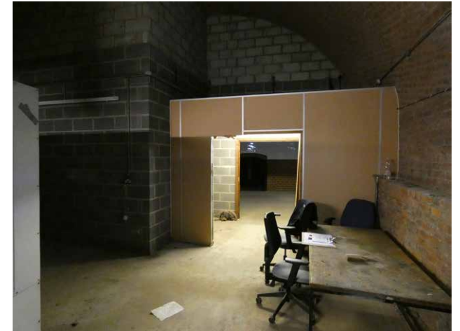
3.28 1830 Viaduct, Arch 2B (Install)
