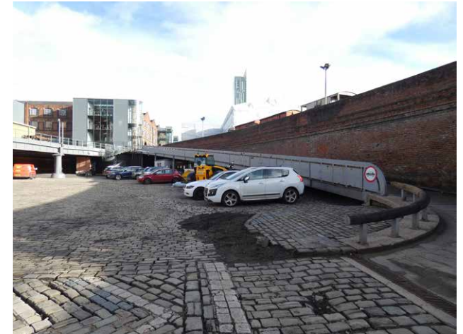
3.3 Outer wall of the 1830 Viaduct and Car Ramp (Insalls)
