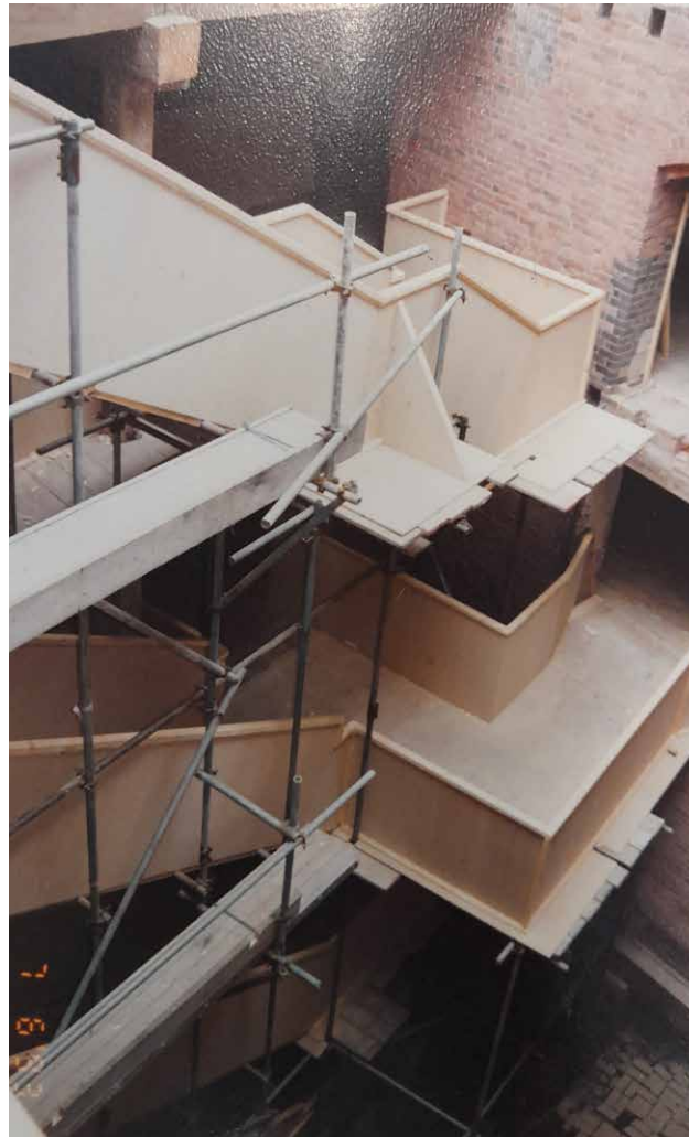
2.13 Insertion of stairway in 1830 Warehouse (SIM Archive 2015-2002).
