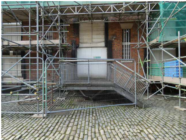
3.14 North elevation, Bay 2 (Insall)
