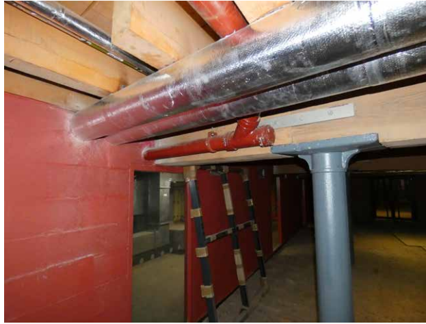
3.23 1830 Warehouse, LG02, blockwork wall to P01 (Insall)
