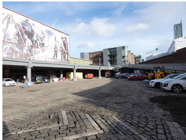
3.5 View of the 1867 Viaduct from the Lower Yard (Insall)
