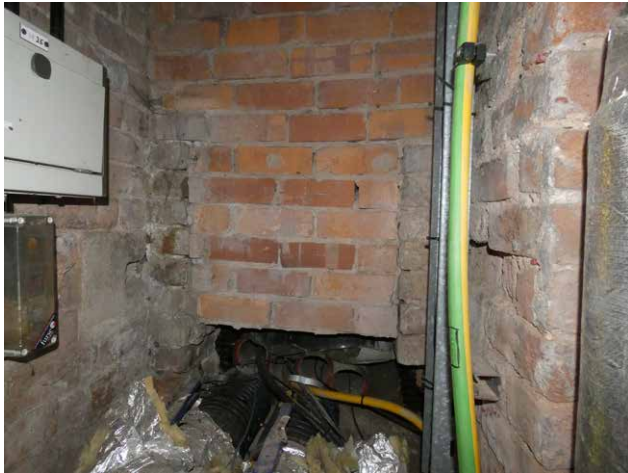
3.22 1830 Warehouse, P01, north wall (Insall)
