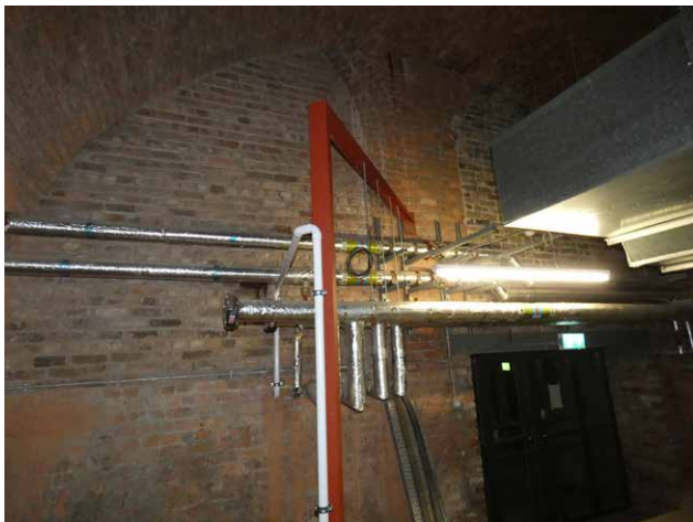
3.29 1830 Viaduct, Arch 2B, north wall (Install)
