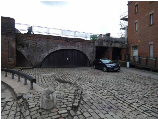
3.4 Concrete bridge of 1830 Viaduct, 1830 Warehouse to right (Insalls)
