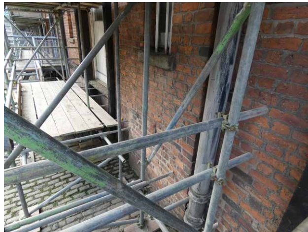
3.15 North elevation, Bay 2 (Insall)
