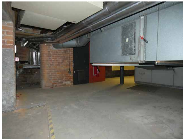
3.20 1830 Warehouse, P01 looking to north wall (Insall)
