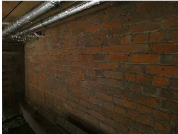
3.25 1830 Warehouse, LG02, south wall lining 1830 Viaduct (Insall)
