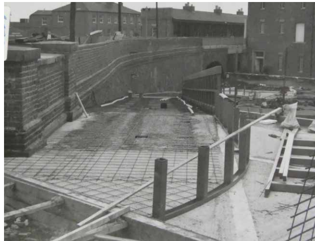
2.19 Construction of the car ramp (SIM Archive YA 2007.41).
