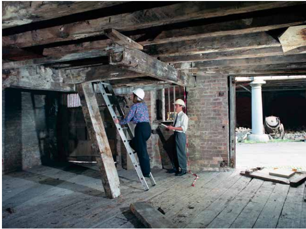
2.12 1830 Warehouse, interior, Aug 1991 (SIM Archive M1703012)
