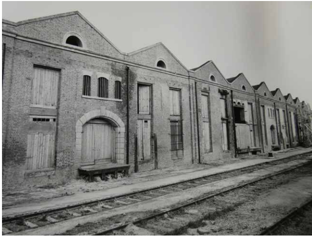
2.9 South elevation of the 1830 Warehouse, c.1979 (SIM Archive 2015-2002).
