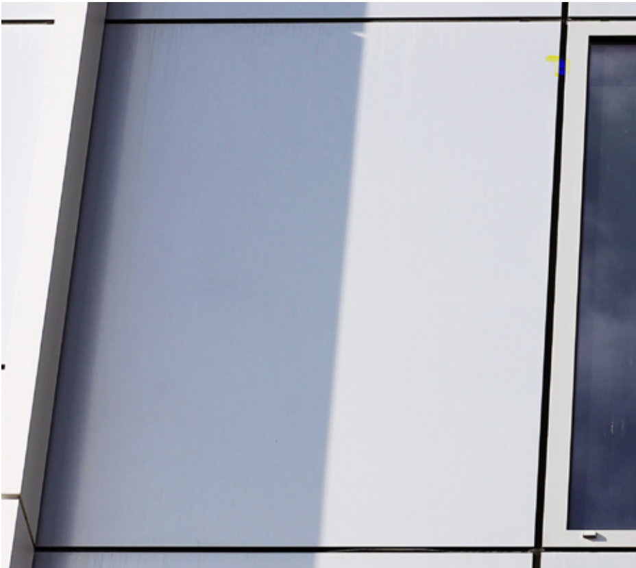
Figure 6: Standard black gaskets between facade panels
