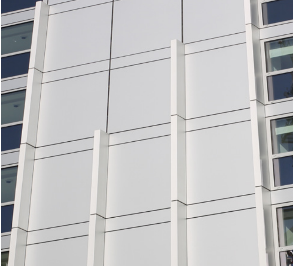
Figure 2: Trinity Riverview cladding panel finish
