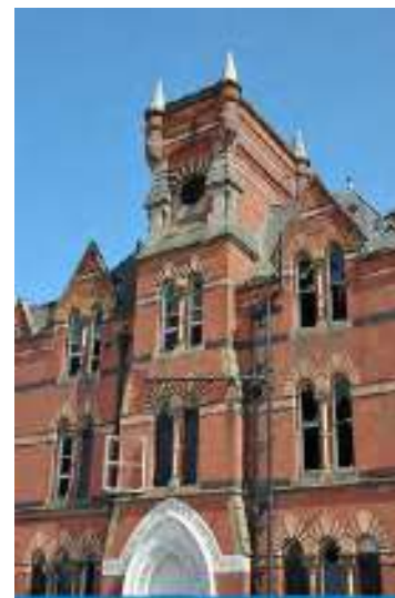
The central tower before its removal and the erection of scaffolding
