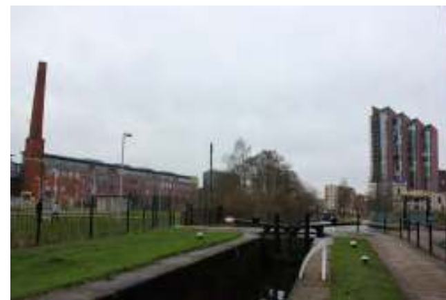
Ashton Canal No. 3 Lock, Listed Grade II
