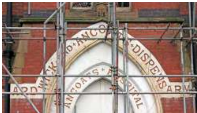
The main entrance of the Ancoats Dispensary has become a symbol of the campaign to save the dispensary.
