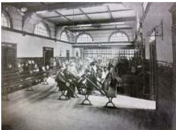
The out-patient's waiting room as it appeared soon after construction, Report of the Committee of the Ardwick and Ancoats Dispensary, 1902, p.4 [Manchester Library, Information and Archives, M325/112]
