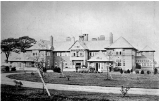
The new convalescent home for Ancoats Hospital patients, opened in 1904, Report of the Committee of the Ardwick and Ancoats Dispensary, 1904, p.49-50 [Manchester Library, Information and Archives M325/112]
