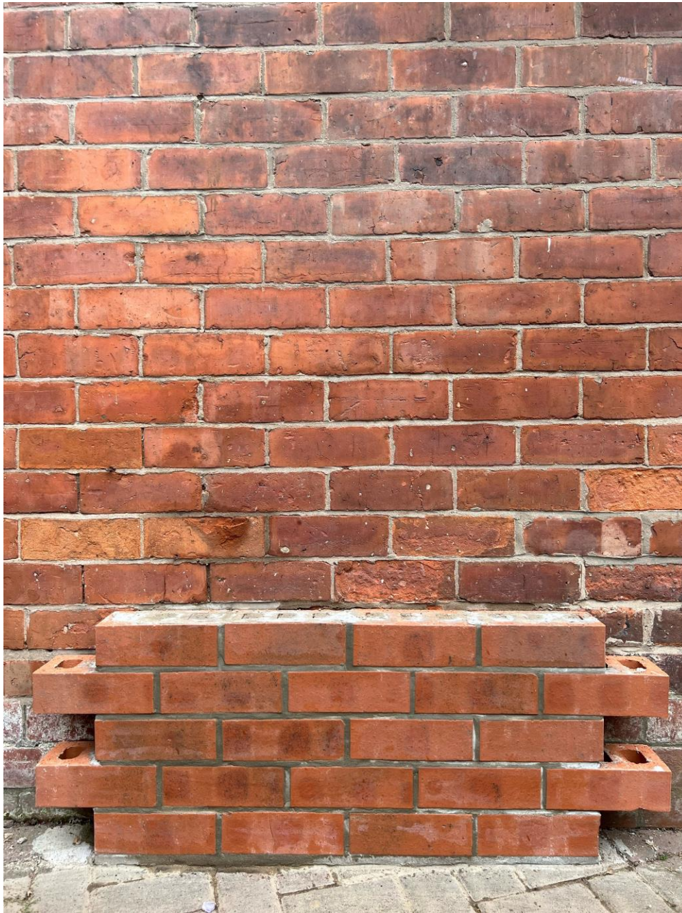
Sample panel of new brick against existing wall
