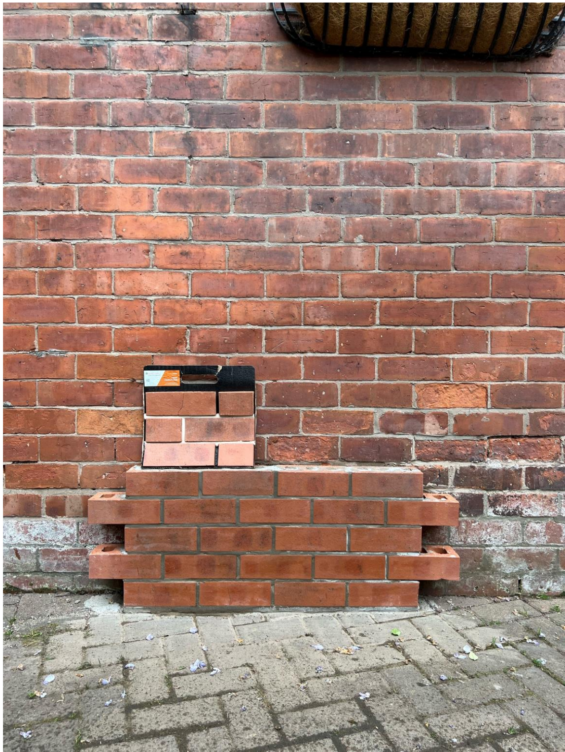
Built sample panel, sample board and existing wall
