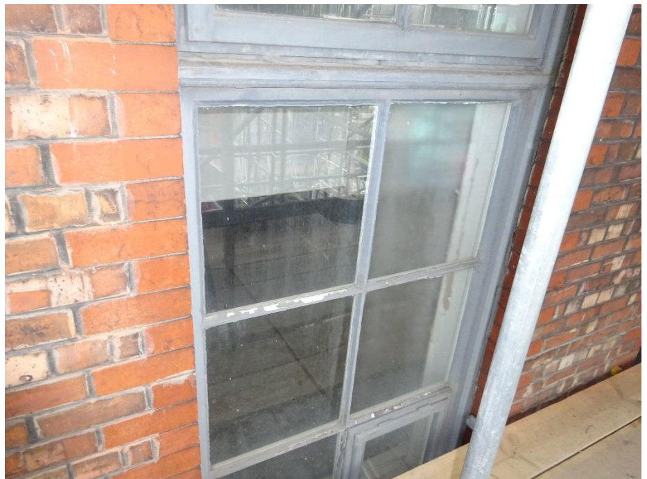
Foam insulation in window frame, South elevation.
