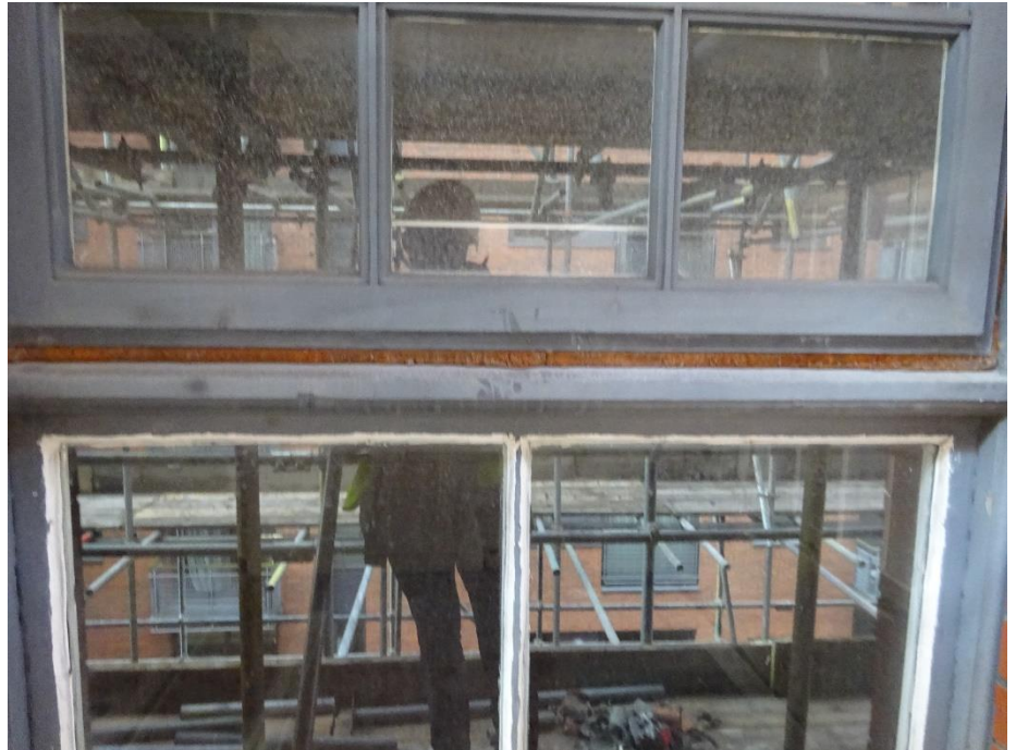
Foam insulation in window frame, East elevation.
