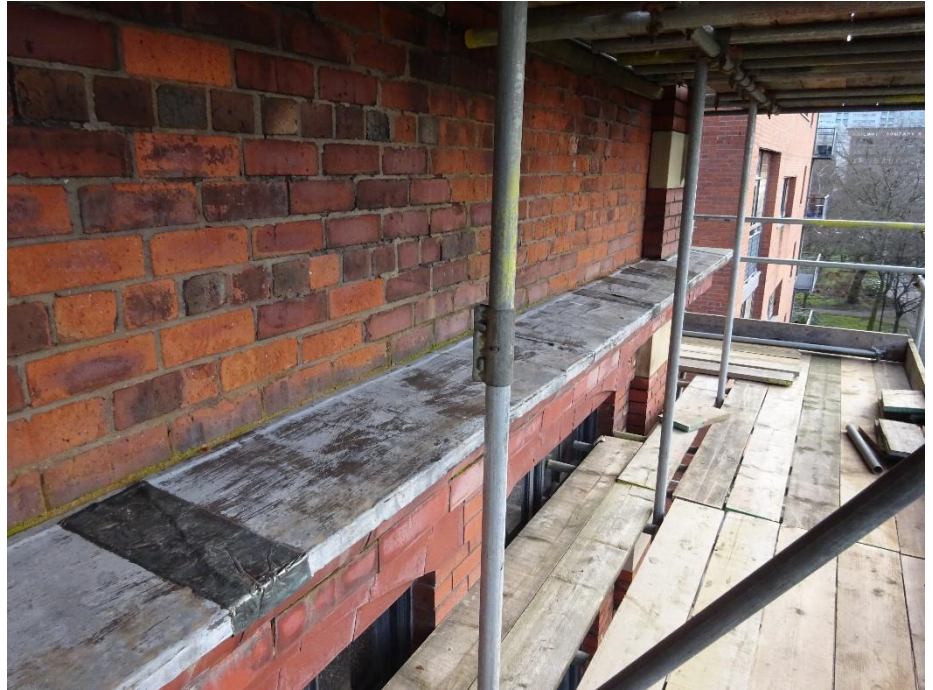
View of patch repairs to the lead projecting cornice to the South elevation.
