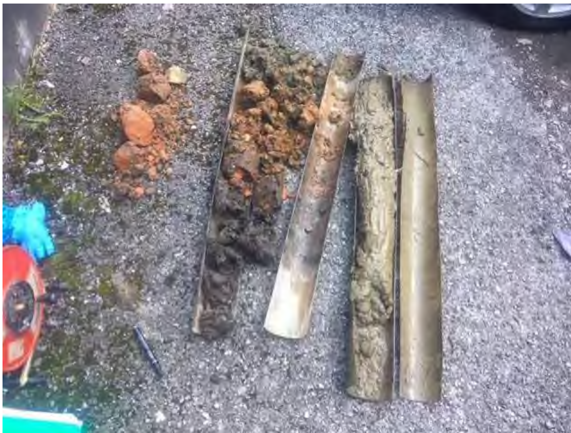
Photograph 5: Arisings from WS1 (1-4mbgl)
