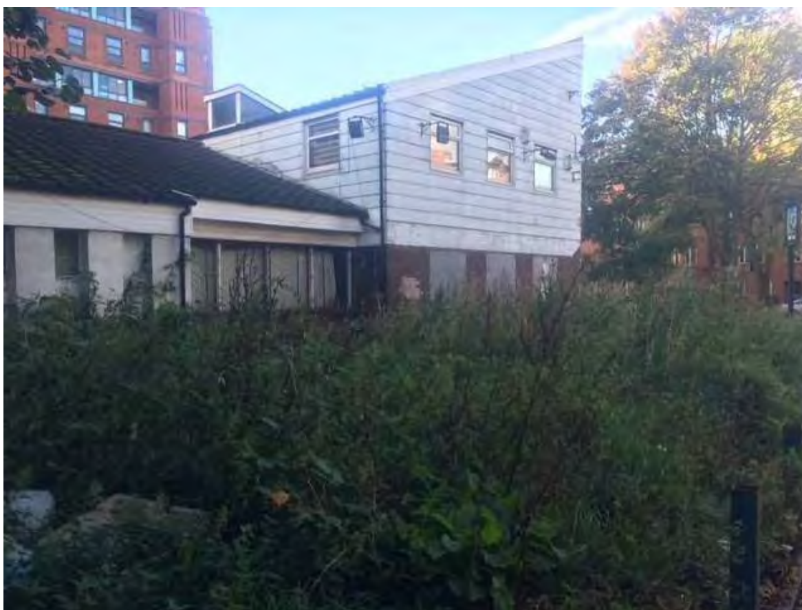
Photograph 2: View of the back of the public house, facing south-west.
