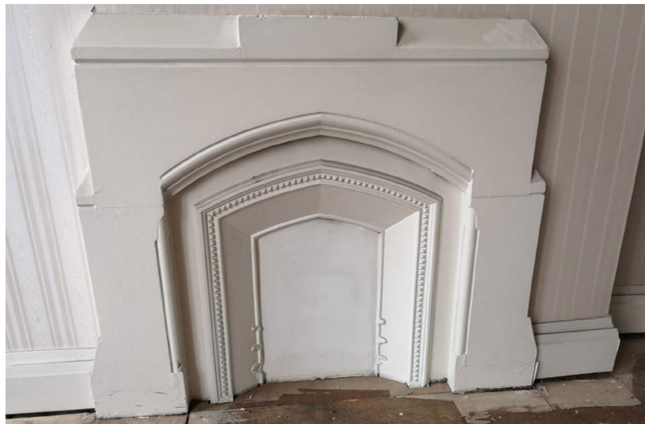
Existing fireplace within southern first floor office area
