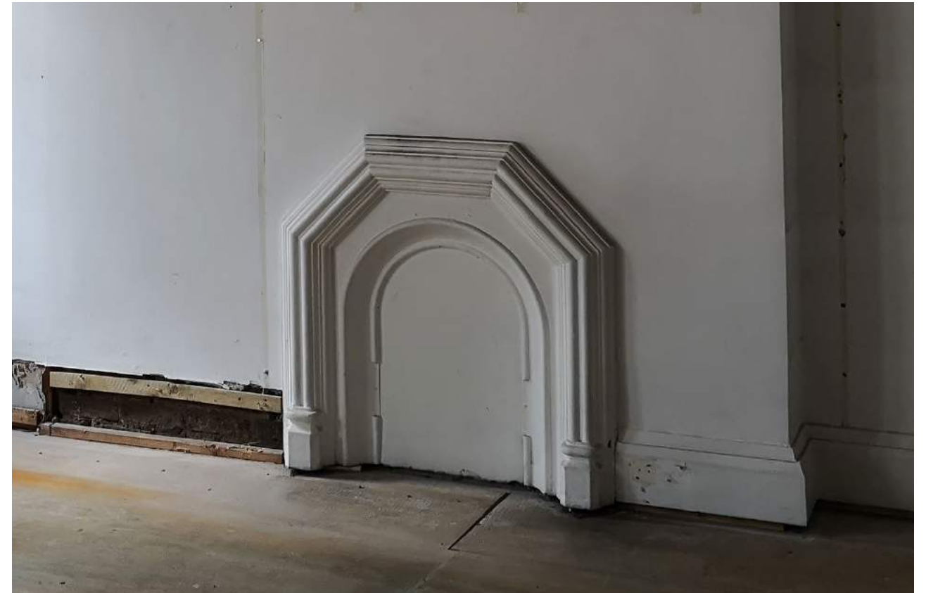
Existing fireplace within southern second floor office area
