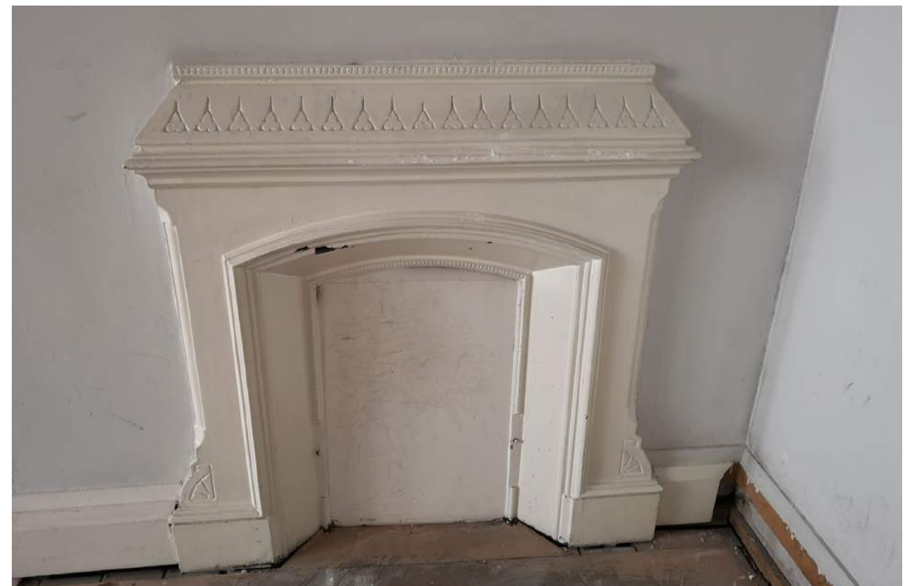
Existing fireplace within southern first floor office area
