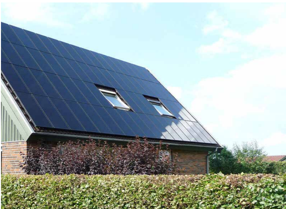
AVANCIS PowerMax unit in use on a residential scheme
