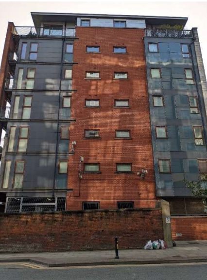
NW Elevation from Ducie Street
