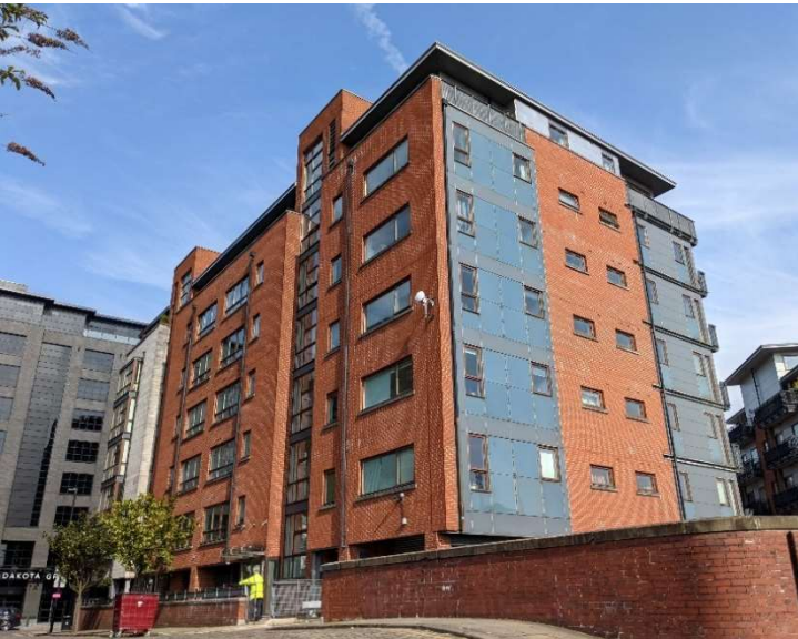
SW & SE Elevation from Jutland Street
