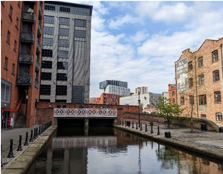
1. View from the footbridge looking north
