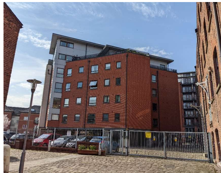
North Elevation (partial) from Junction Works/The Stables
