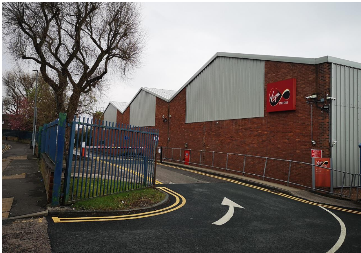
View from Timpson Road of the Virgin Media buildings showing roof profile
