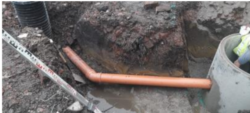
Photographs of private foul water drainage inspection chambers at a very early (L) and then more advanced (R) stage of construction. Constructed in accordance with Carley Daines and Partners drawings and building regulations Document H.
