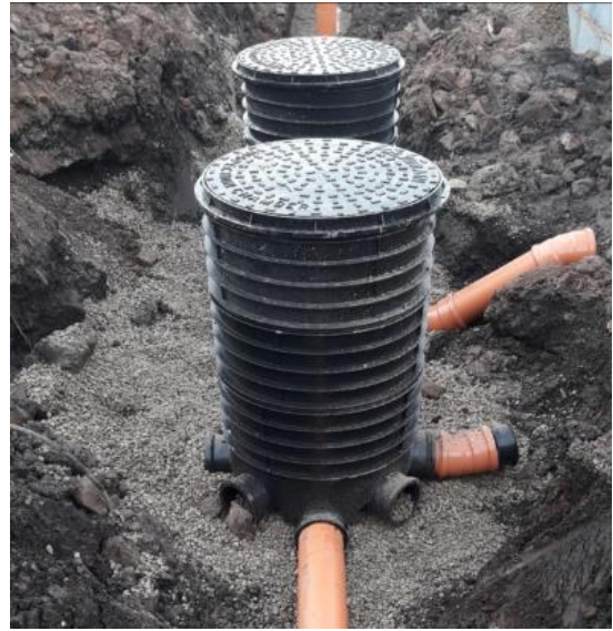
Photographs of private foul water drainage inspection chambers at a very early (L) and then more advanced (R) stage of construction. Constructed in accordance with Carley Daines and Partners drawings and building regulations Document H.
