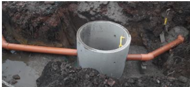
Photographs showing the construction of the flow control chamber MH S14 and its' connection to the combined system confirm drainage was laid in accordance with Building Regulations Document H, and Hydro International design drawing. Also per the detailed construction design shown on Carley Daines and Partners drawings.
