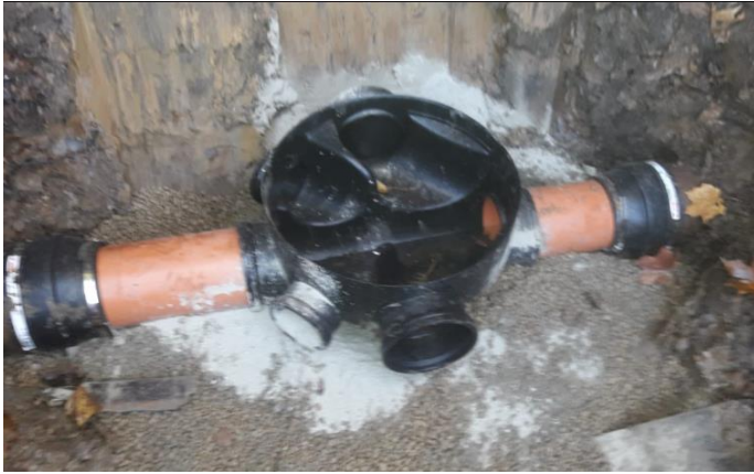
Photographs of private foul water drainage inspection chambers at a very early (L) and then more advanced (R) stage of construction. Constructed in accordance with Carley Daines and Partners drawings and building regulations Document H.
