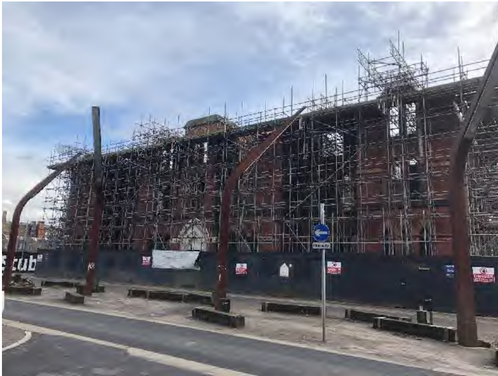
Figure 21: View from Old Mill Street
