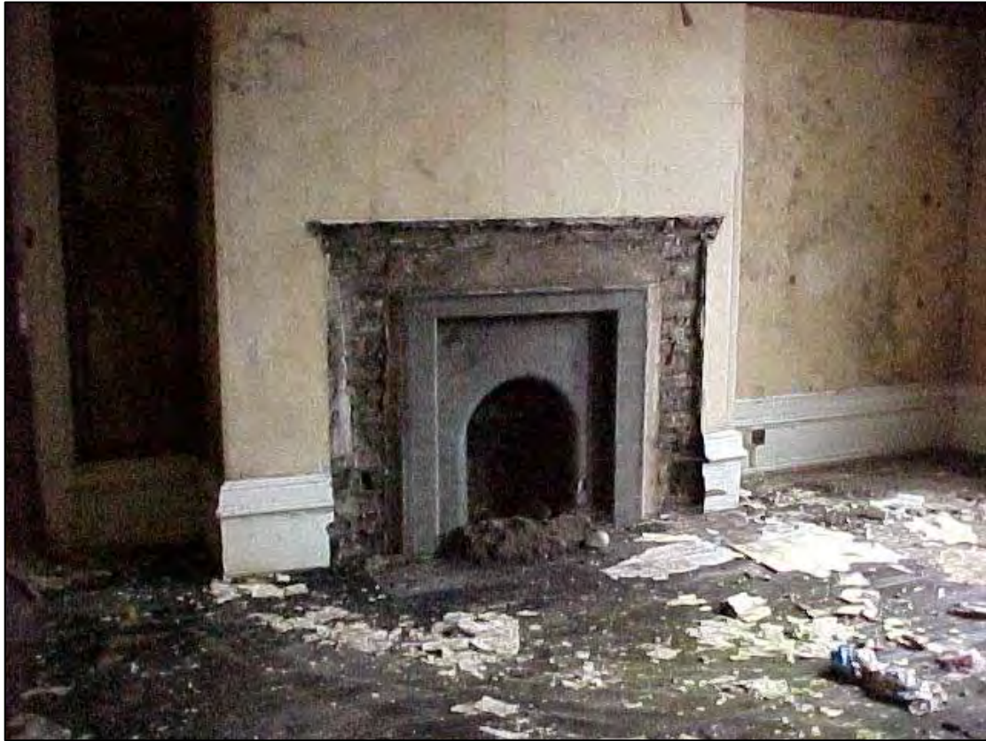
Plate 21: Fireplace in the 'panelled' office
