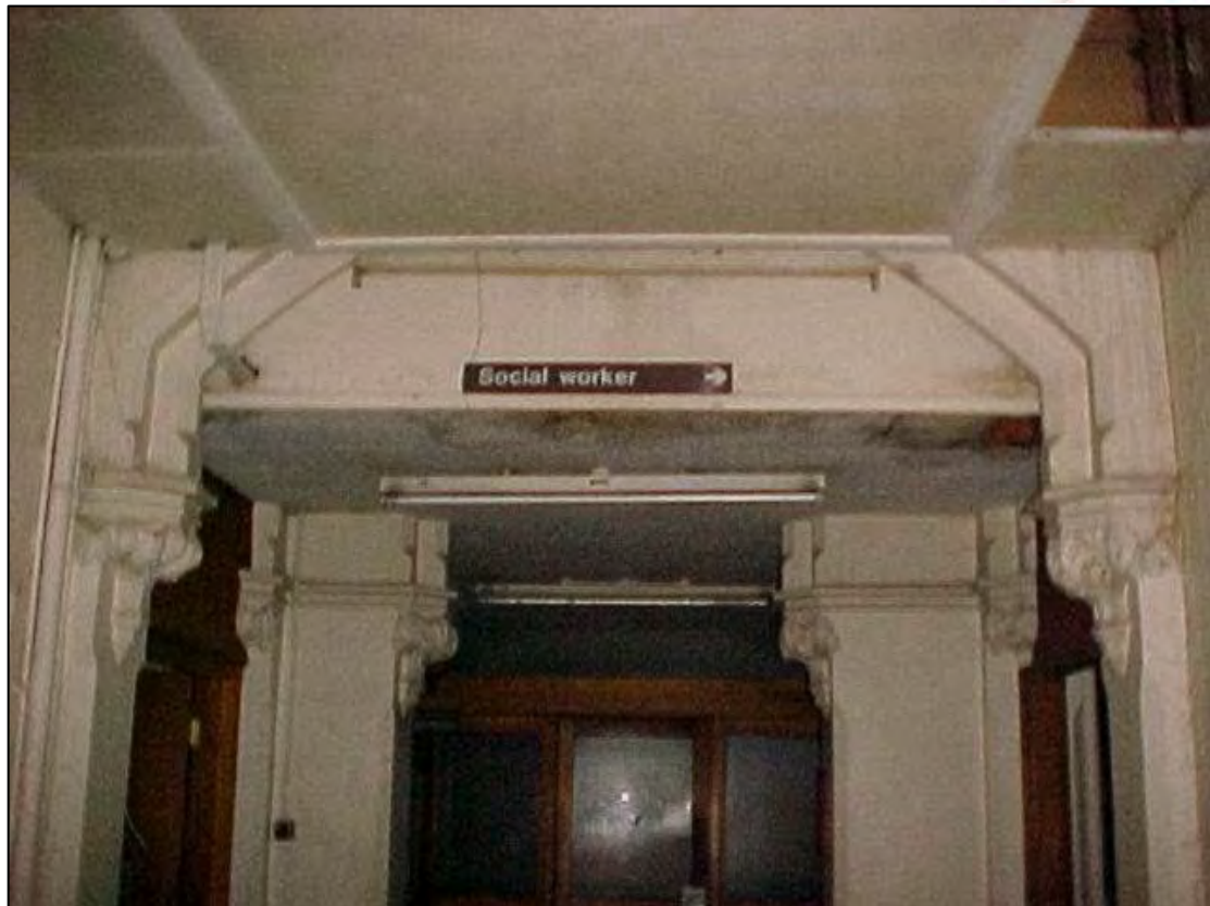
Plate 23: Decorative archway to the principal Old Mill Street entrance
