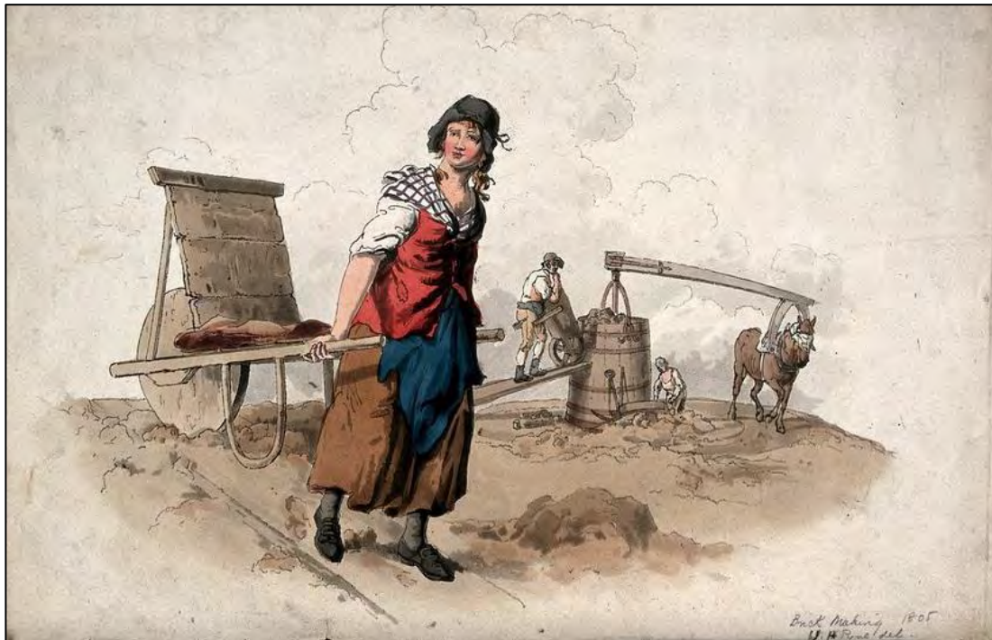
Plate 7: Brickmaking illustration, by William Pyne, showing a young woman taking clay to a vat and a horse in the background powering a stirring mechanism to mix the clay before it is shaped into bricks
