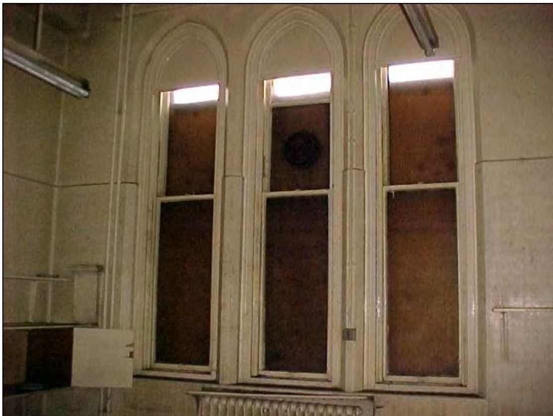
Plate 20: Triple neo-gothic windows in an office at western elevation second storey
