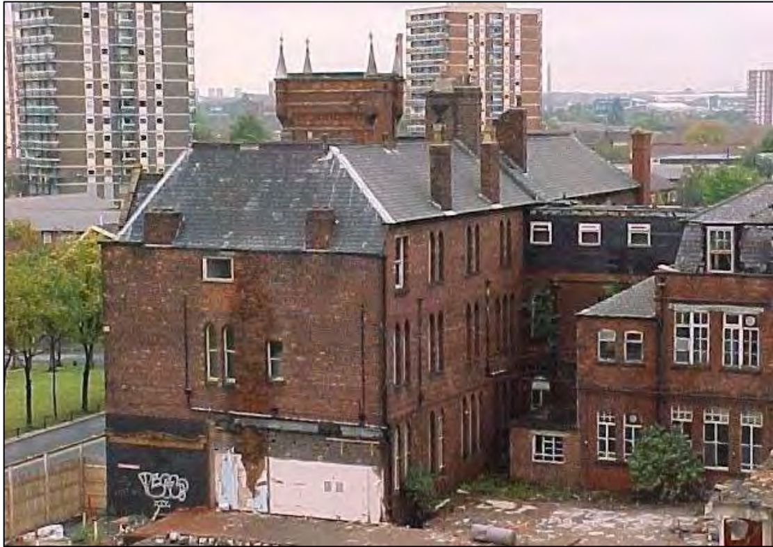
Plate 19: General view of the Old Hospital (dispensary building) southern elevation looking to Old Mill Street
