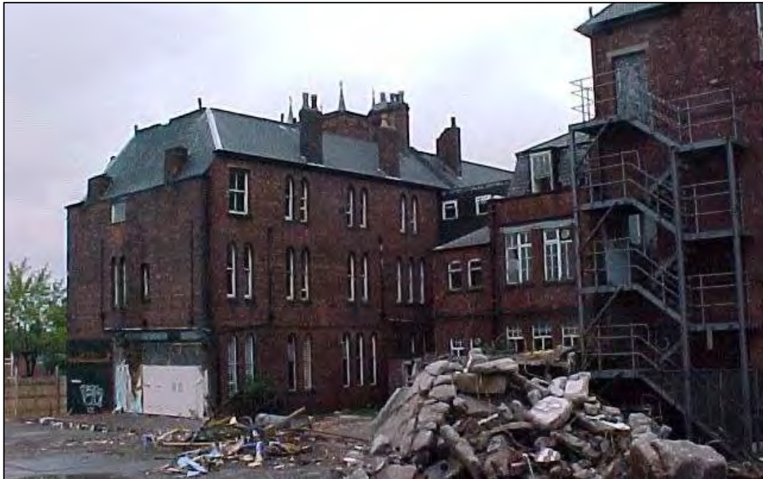
Plate 18: General view between the Old and New hospitals at their eastern and western elevations
