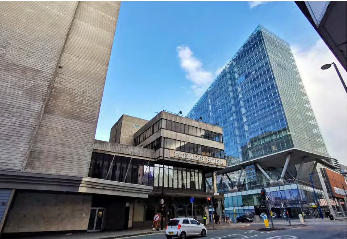
View towards existing Hotel & Premier House entrance
