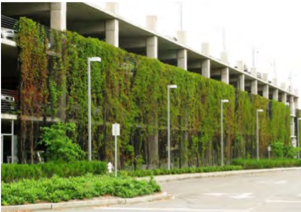
Planting on a concrete backdrop
