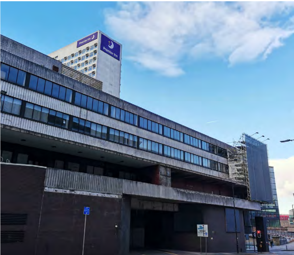
View from Deansgate to existing service yard entrance
