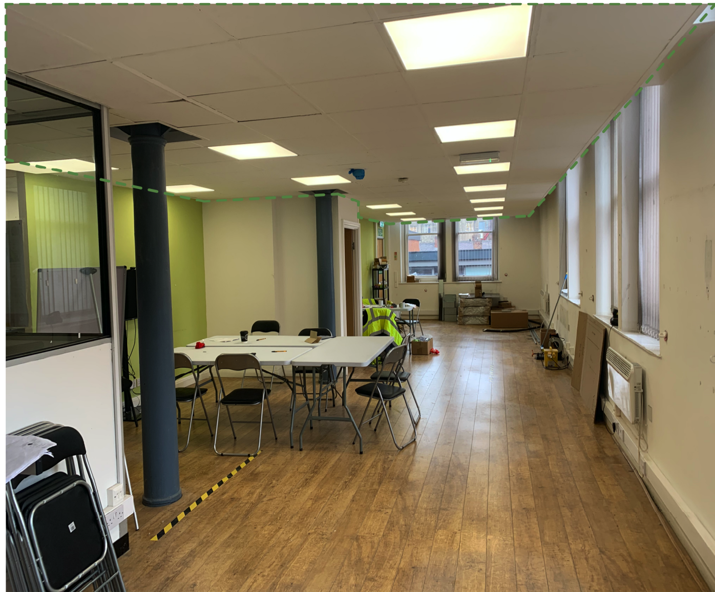
FOURWAYS HOUSE, SECOND FLOOR PHOTOGRAPH SHOWING SUSPENDED CEILINGS
