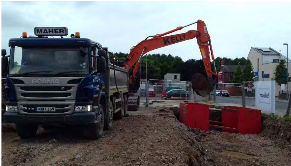
PLATE 1 – EXCAVATION OF SOURCE AREA 1
