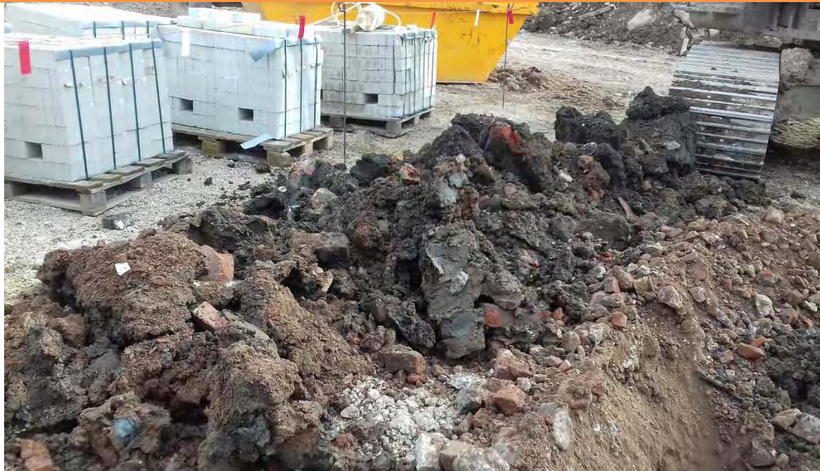
PLATE 26 – ARISINGS OF PRELIMINARY TRIAL PITS
