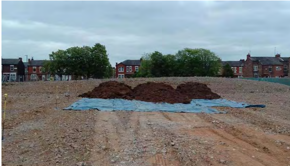
PLATE 3 – STOCKPILING OF EXCAVATED MATERIAL FROM SOURCE AREA 1
