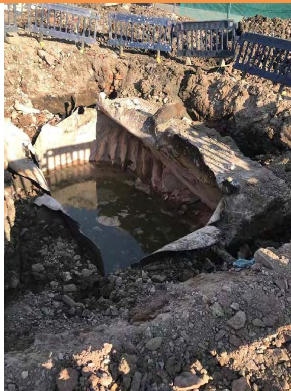
PLATE 32 – IN SITU UNDERGROUND TANK BENEATH FORMER SUBSTATION
