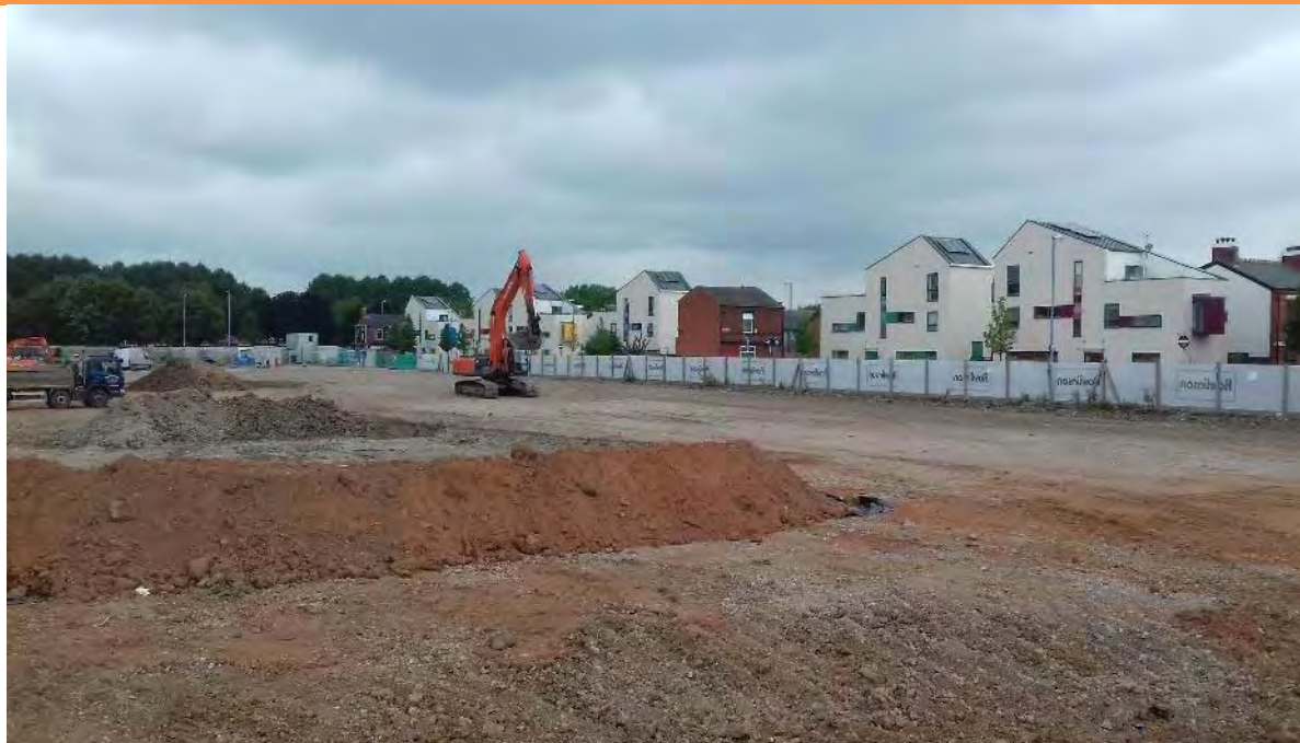
PLATE 22 – WEST OF SITE
