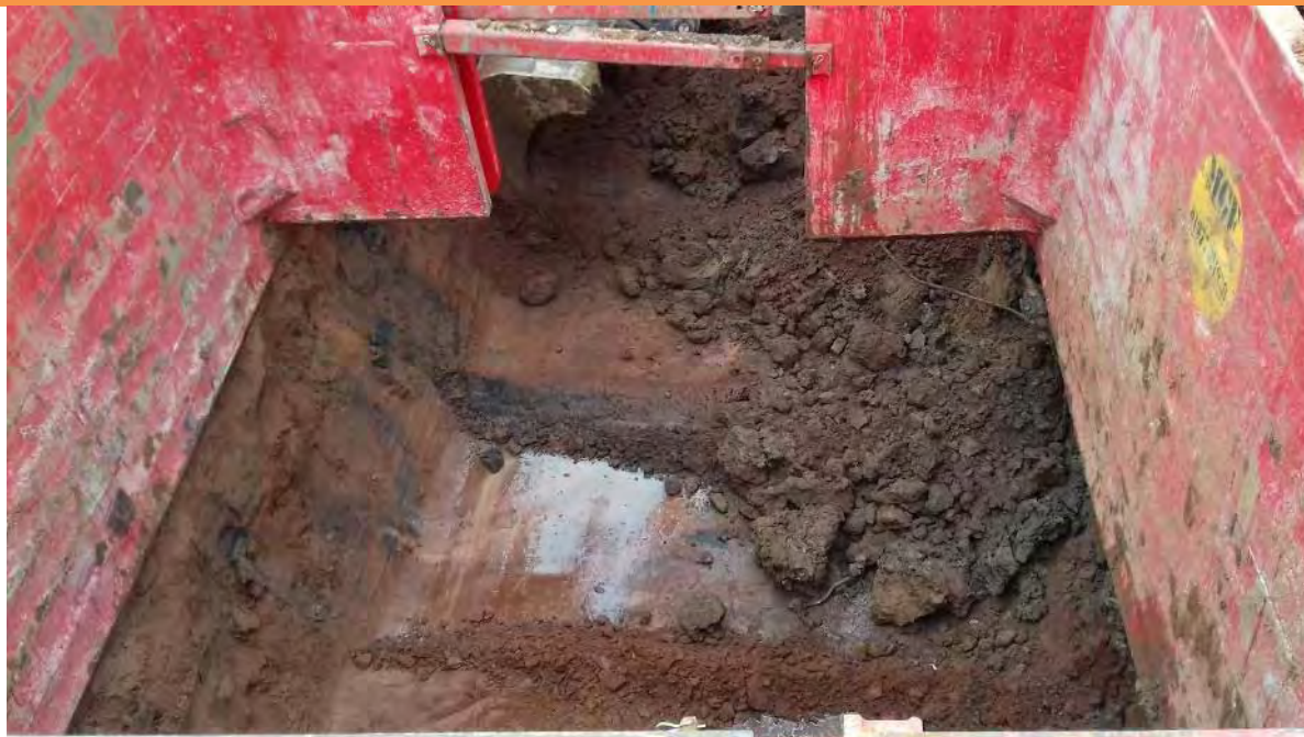
PLATE 5 – BASE OF SOURCE AREA 1 AFTER EXCAVATION
