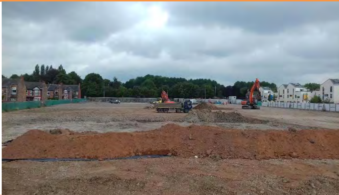
PLATE 21 – VIEW OF WEST OF SITE
