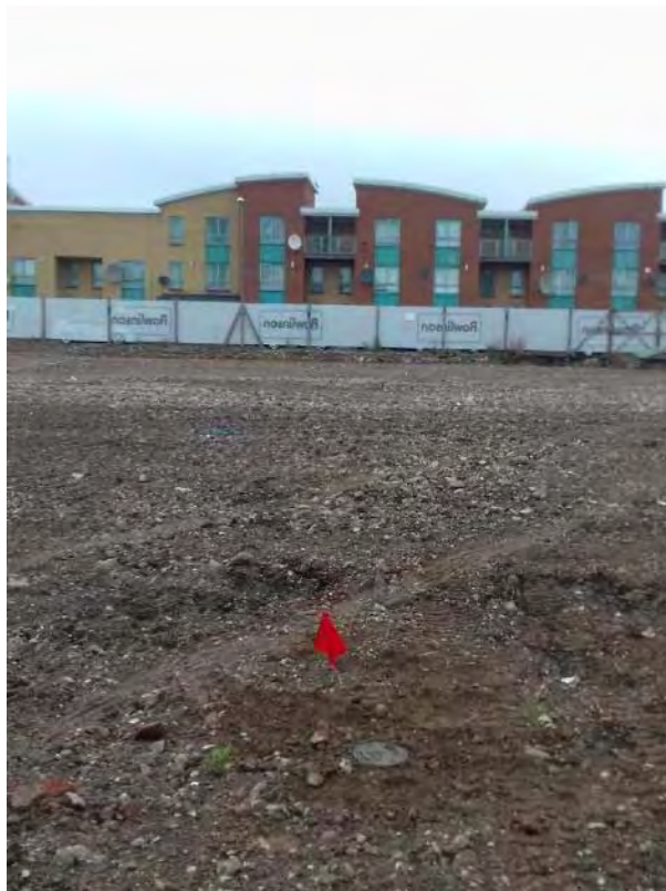
PLATE 12 –INSTALLED VAPOUR RISK ASSESSMENT BOREHOLES
