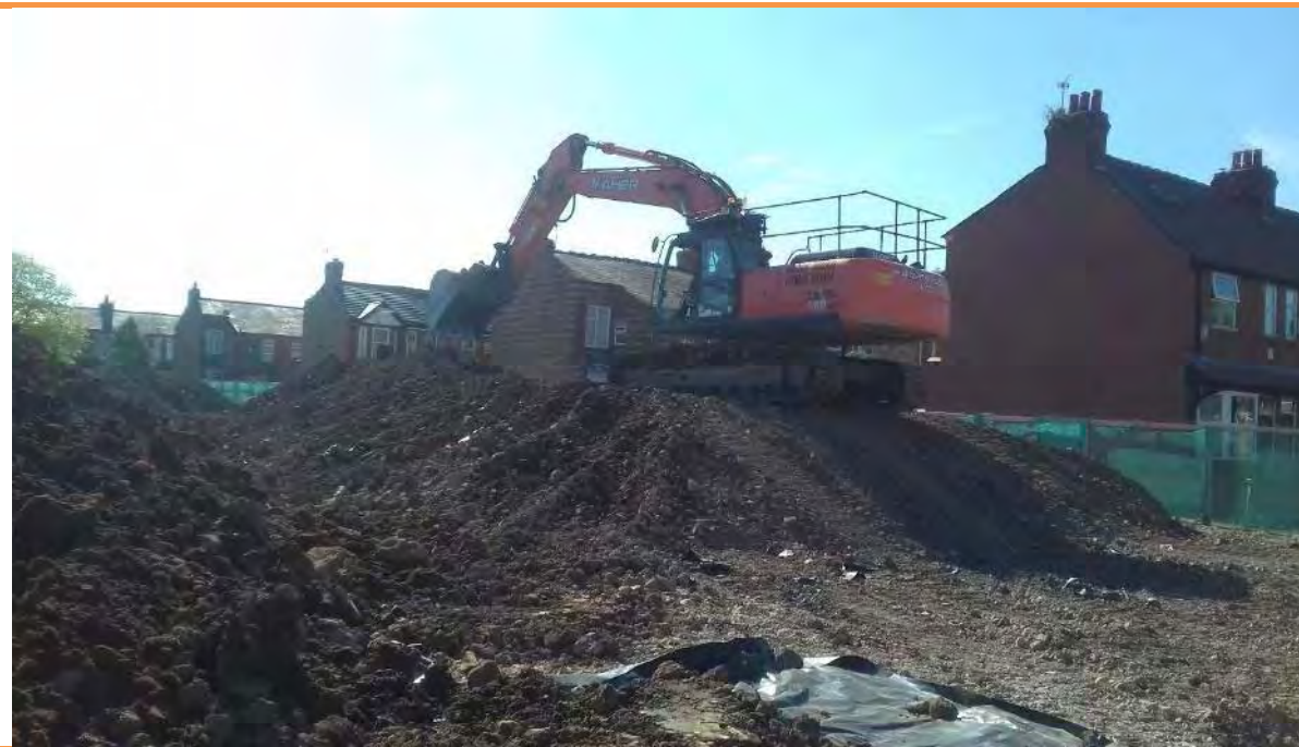
PLATE 9 – CONTAMINATED MATERIAL BEING TURNED
