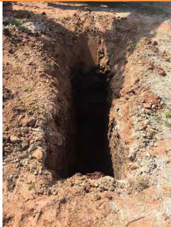
PLATE 14 – SOURCE AREA 2 FURTHER INVESTIGATION TRIAL PIT
