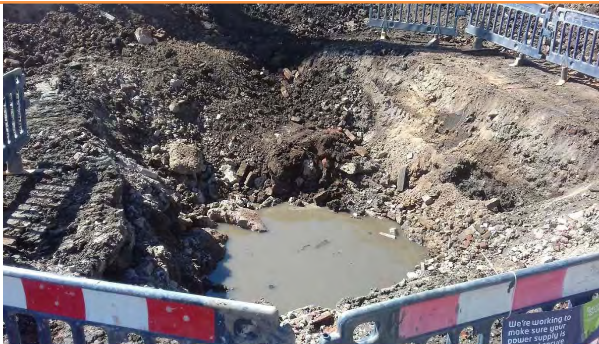
PLATE 28 – POST DEMOLITION EXCAVATION BENEATH SUBSTATION
