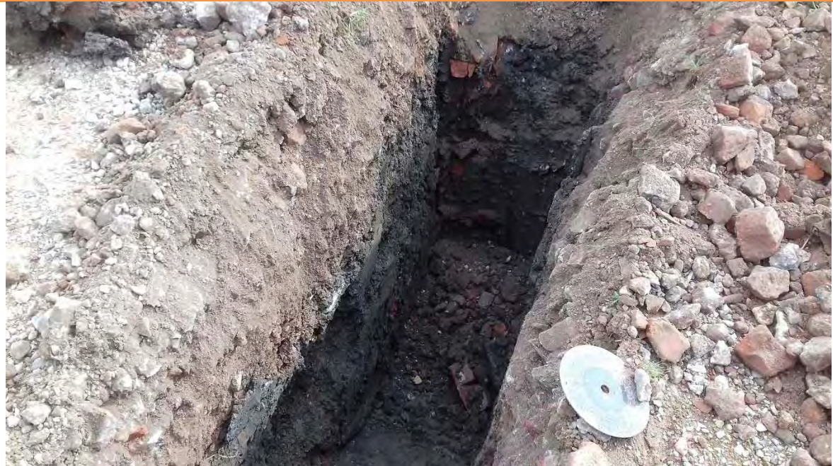
PLATE 25 – PRELIMINARY TRIAL PITS IN VINICITY OF SUBSTATION
