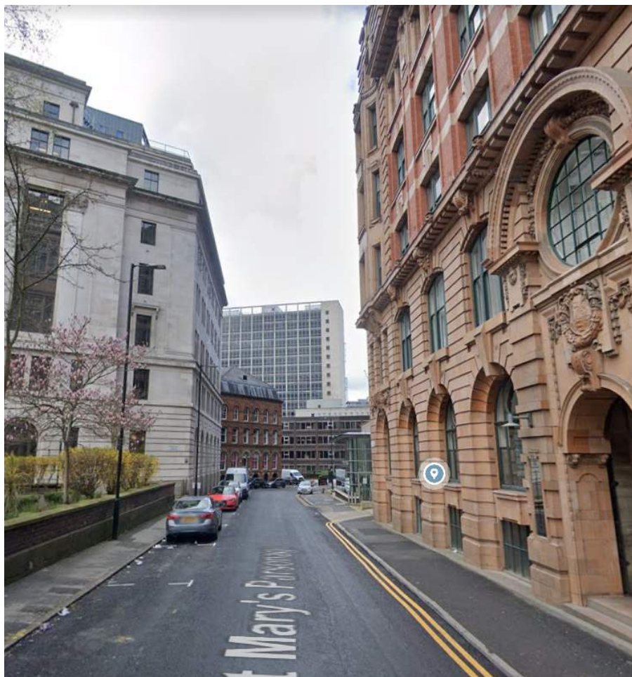
Figure 4: Photo taken from outside the National Building westbound on St Mary's Parsonage, Alberton House is obscured behind the building and cannot be seen from this area of the conservation area.
