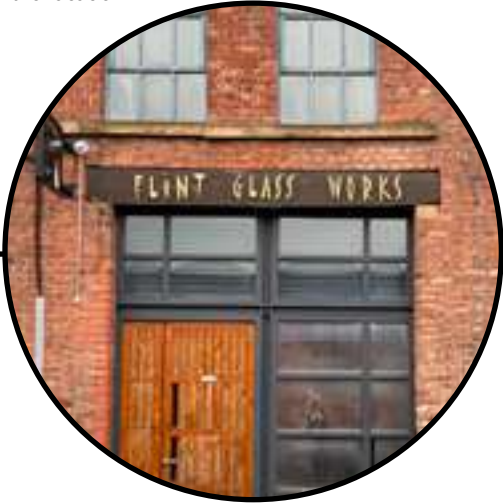
Larger opening bays at ground level.
