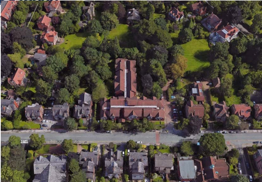
Photo 2. The neighbouring properties on Barlow Moor Road
