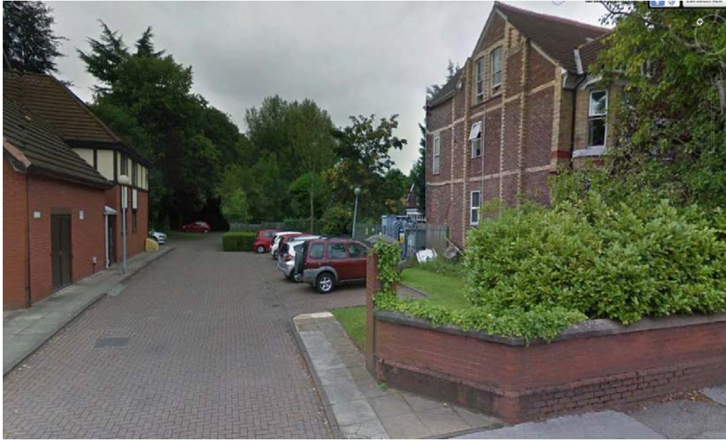
Photo 5. Parkfield Court with neighbouring property to right
