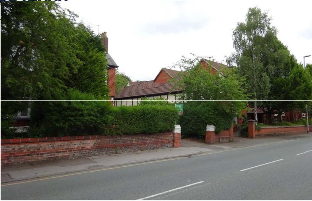
Photo 4. Parkfield Court with neighbouring property to left
