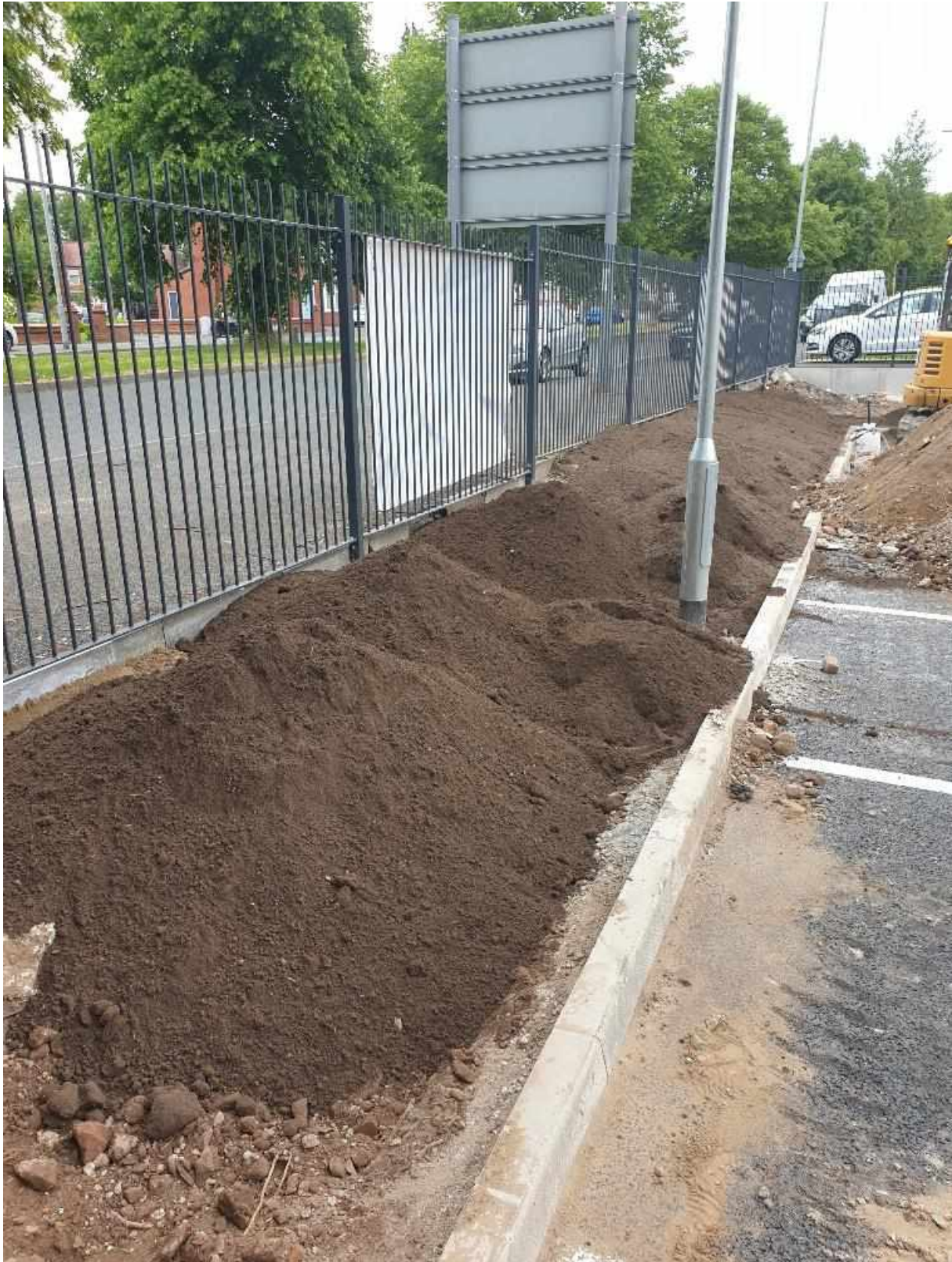
Photograph 6 Reduced area of thickness to the north-west of the car parking on Kingsway due to linear strip, changes in elevation and street furniture.
