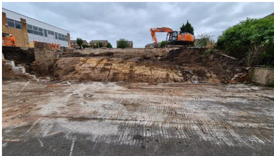
Completed excavation area as shown on drawing JK20-6266-03.
