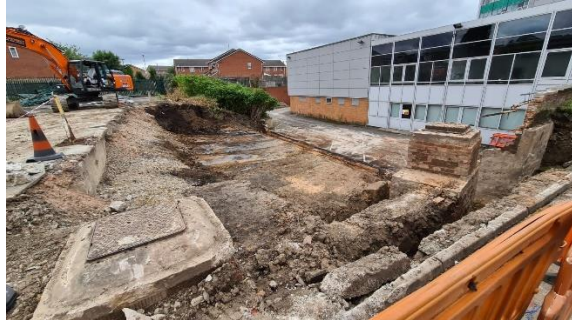
Completed excavation area as shown on drawing JK20-6266-03. Manhole structures and associated pipes left in-situ.
