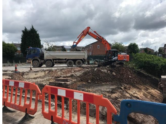
Excavation and loading of tipper wagons with materials containing Japanese knotweed.
