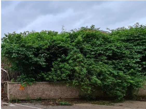
Vegetation within southern section of embankment area left in-situ due to the presence of nesting birds.
