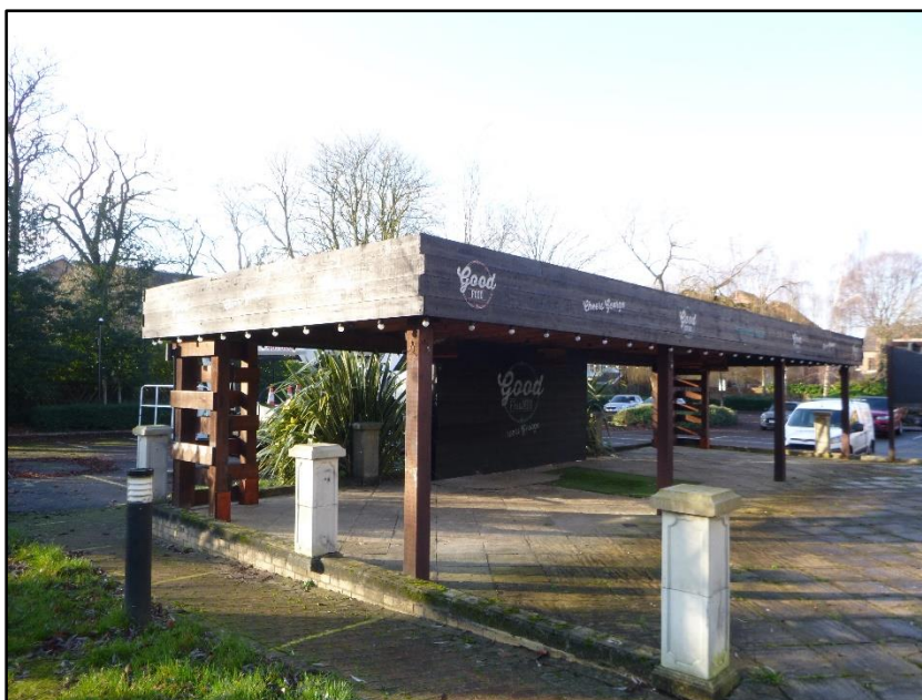
Photograph 13 showing the shelter
