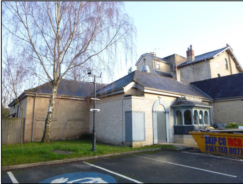
Photograph 8 showing the roof of the property
