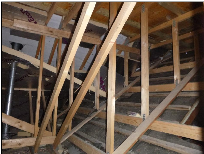
Photograph 10 showing the roof void above north-western extension
