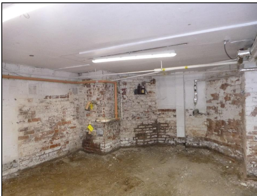
Photograph 12 showing the basement in the main building
