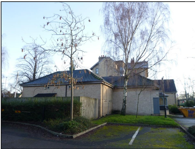
Photograph 7 showing the one-storey extensions
