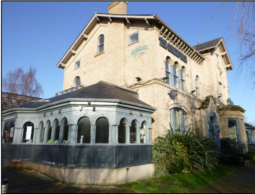
Photograph 6 showing the exterior of the building
