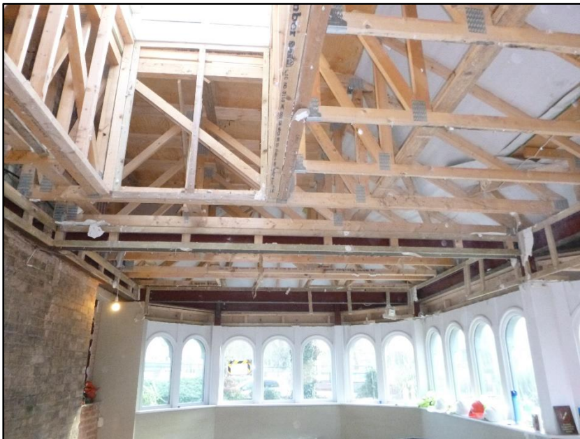
Photograph 9 showing the roof of the conservatory extension
