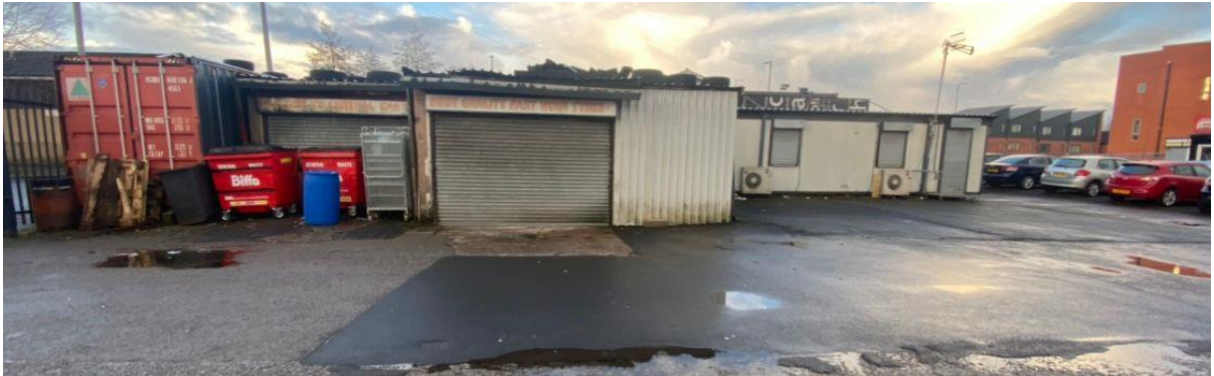
Rear of the structure.
