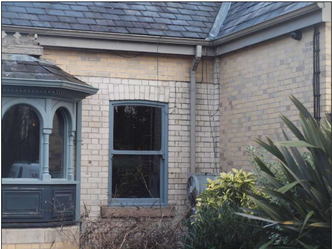
Plate 36: Detail of window and rebuilding
