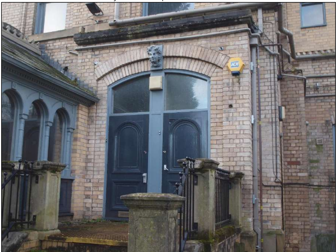
Plate 46: Detail of doorway, formerly a window
