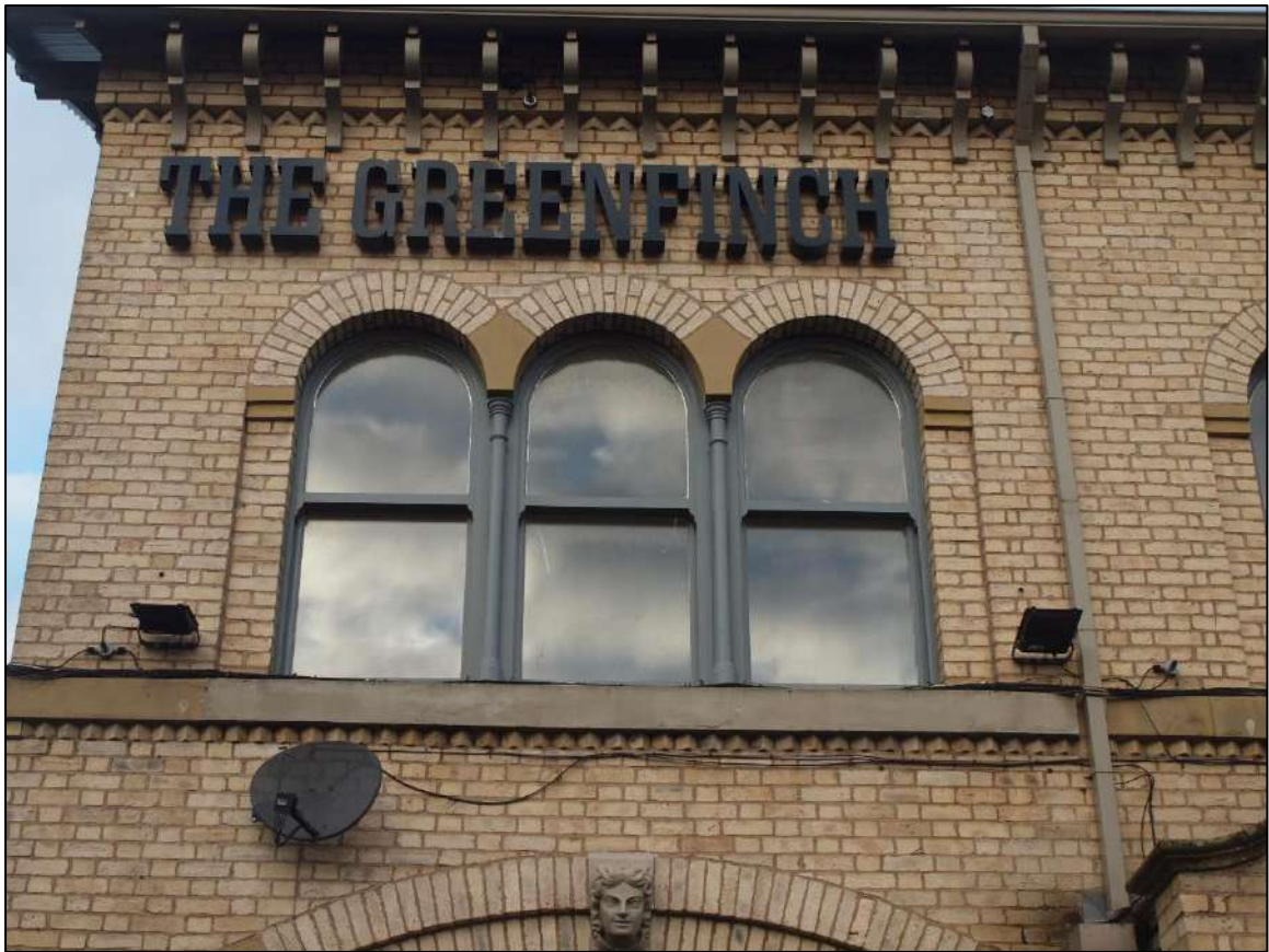
Plate 23: First floor windows above
