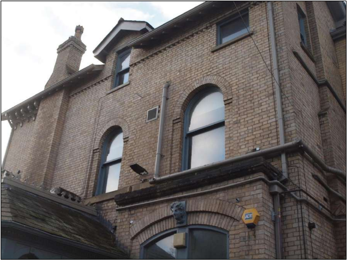
Plate 47: Detail of first and attic floors
