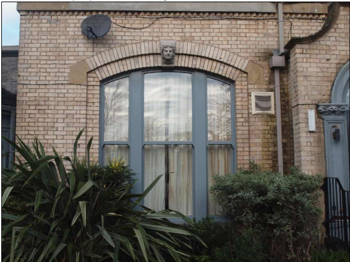
Plate 22: ground floor window in left bay
