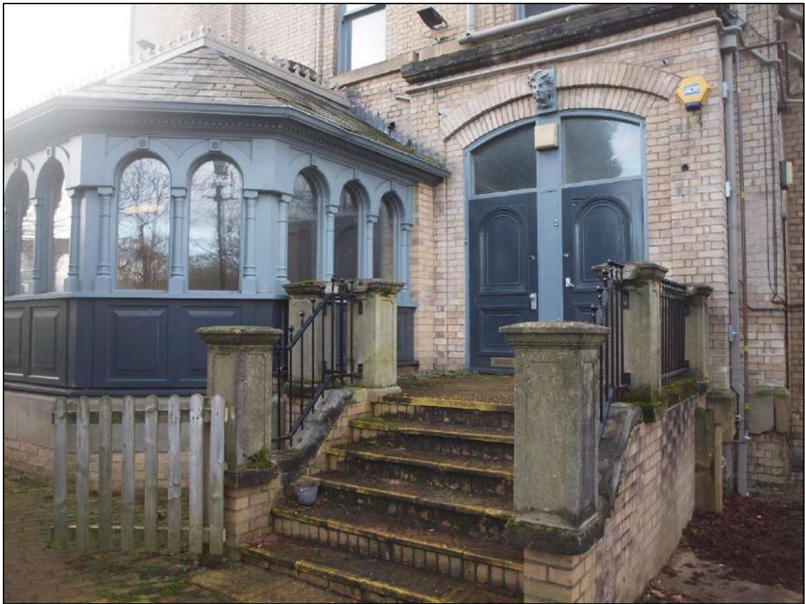
Plate 45: Ground floor doorway with stairs up
