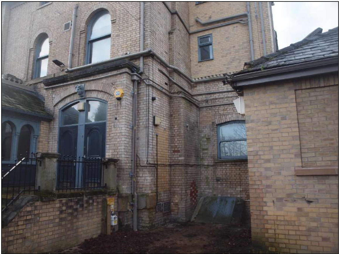
Plate 49: Ground floor rear extension with stair tower over
