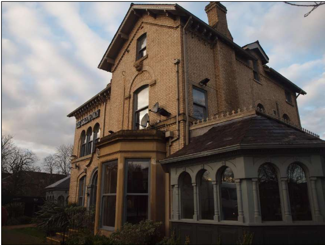
Plate 19: General shot of the southeast elevation
