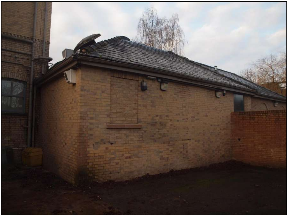
Plate 50: Modern extension to north west
