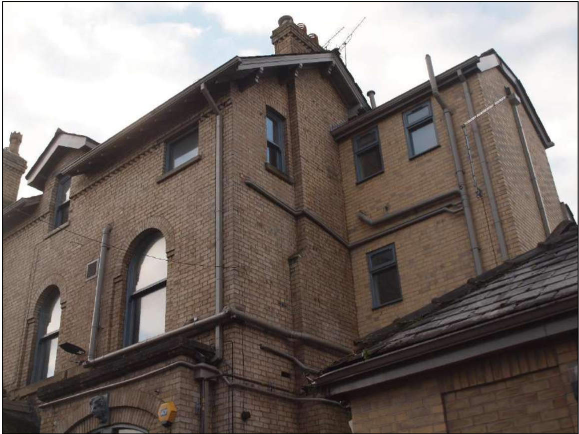
Plate 39: Detail of stair tower
