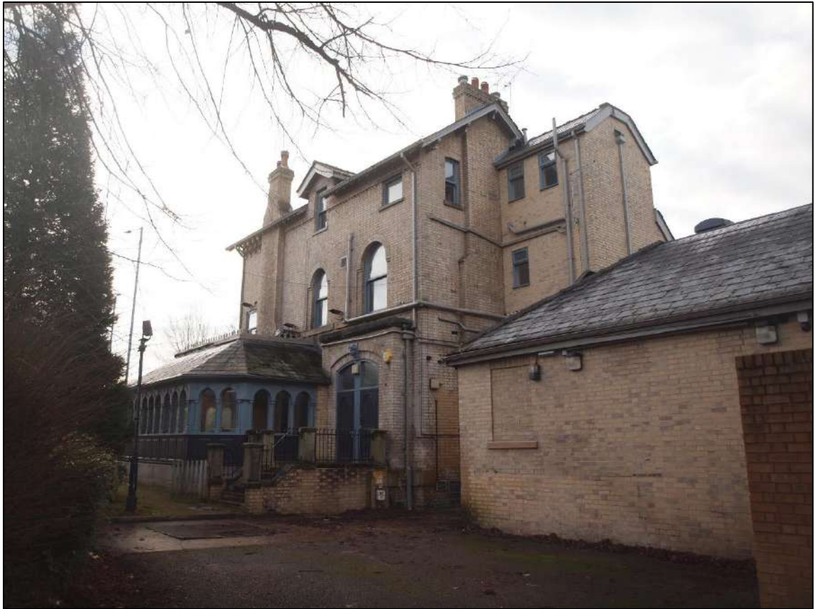
Plate 43: General shot of North east elevation
