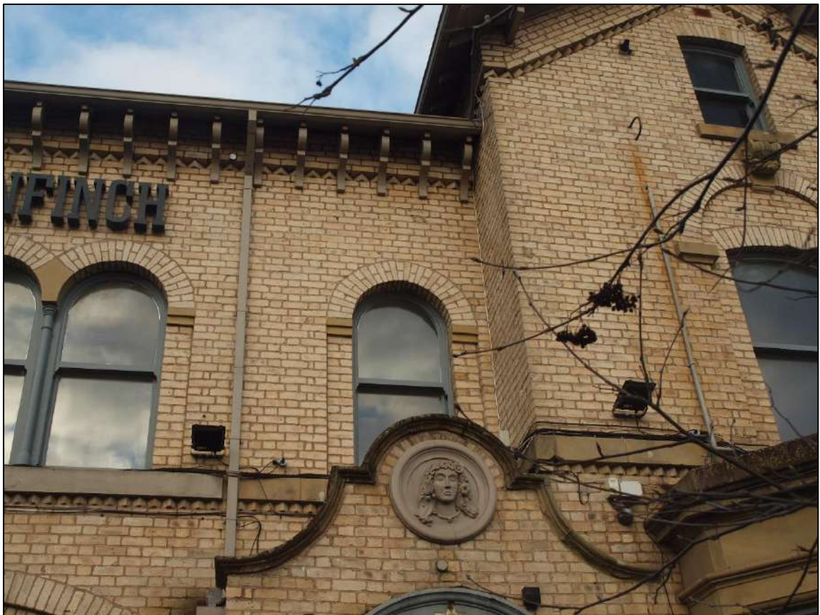
Plate 24: First floor window, central bay
