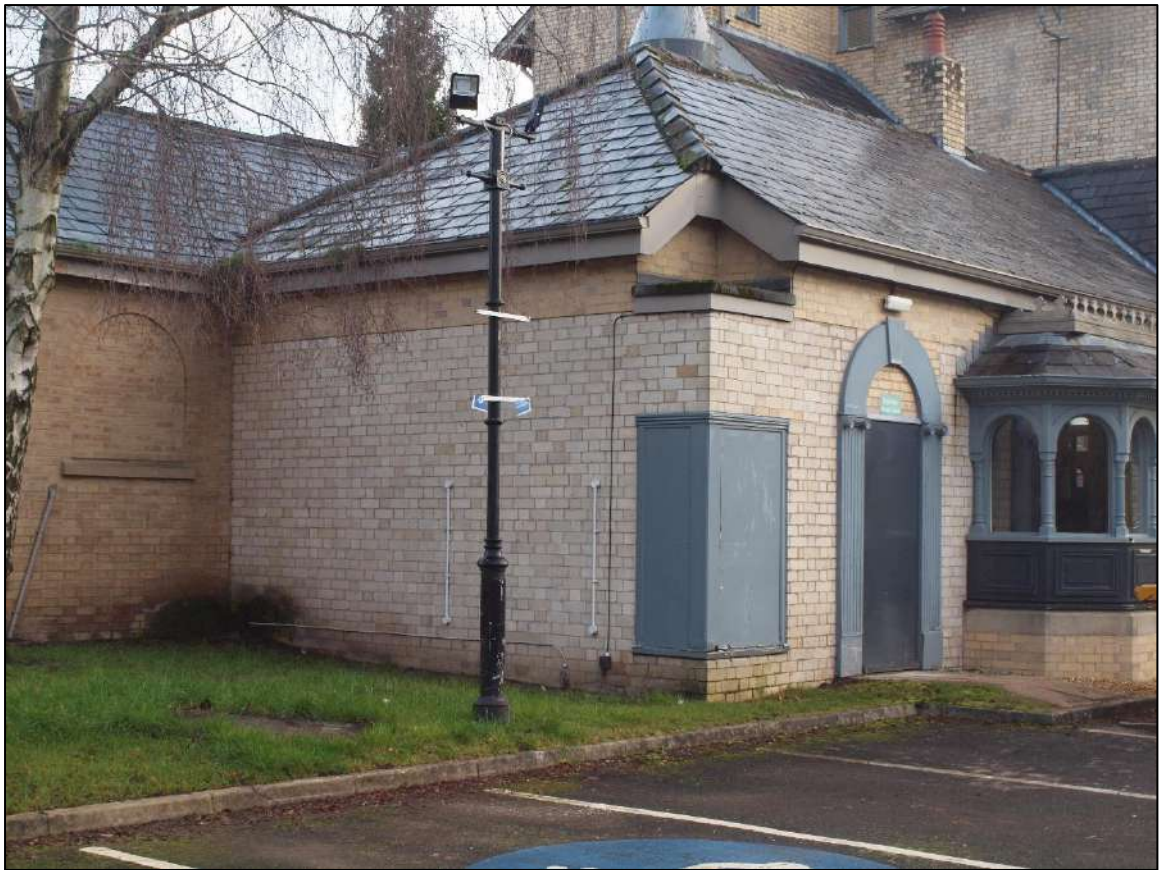
Plate 41: North west elevation of late 19 th century extension
