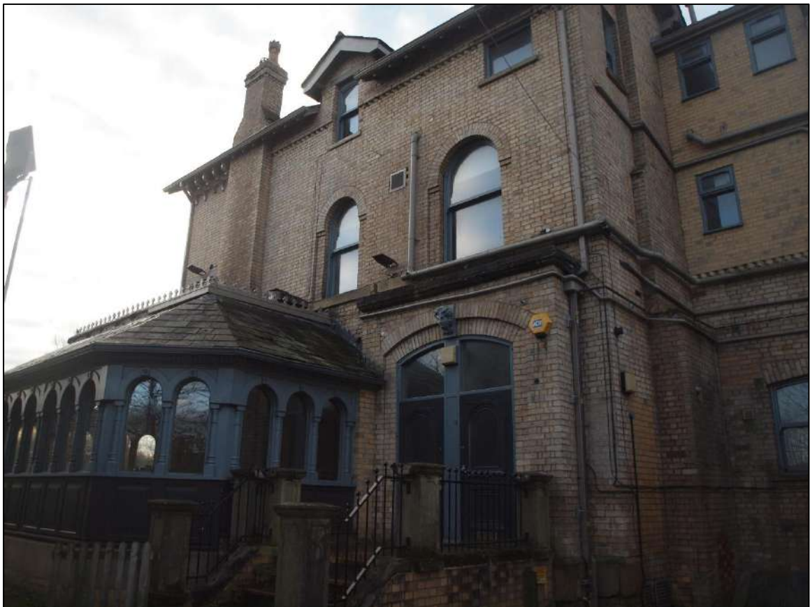
Plate 44: North east elevation of house
