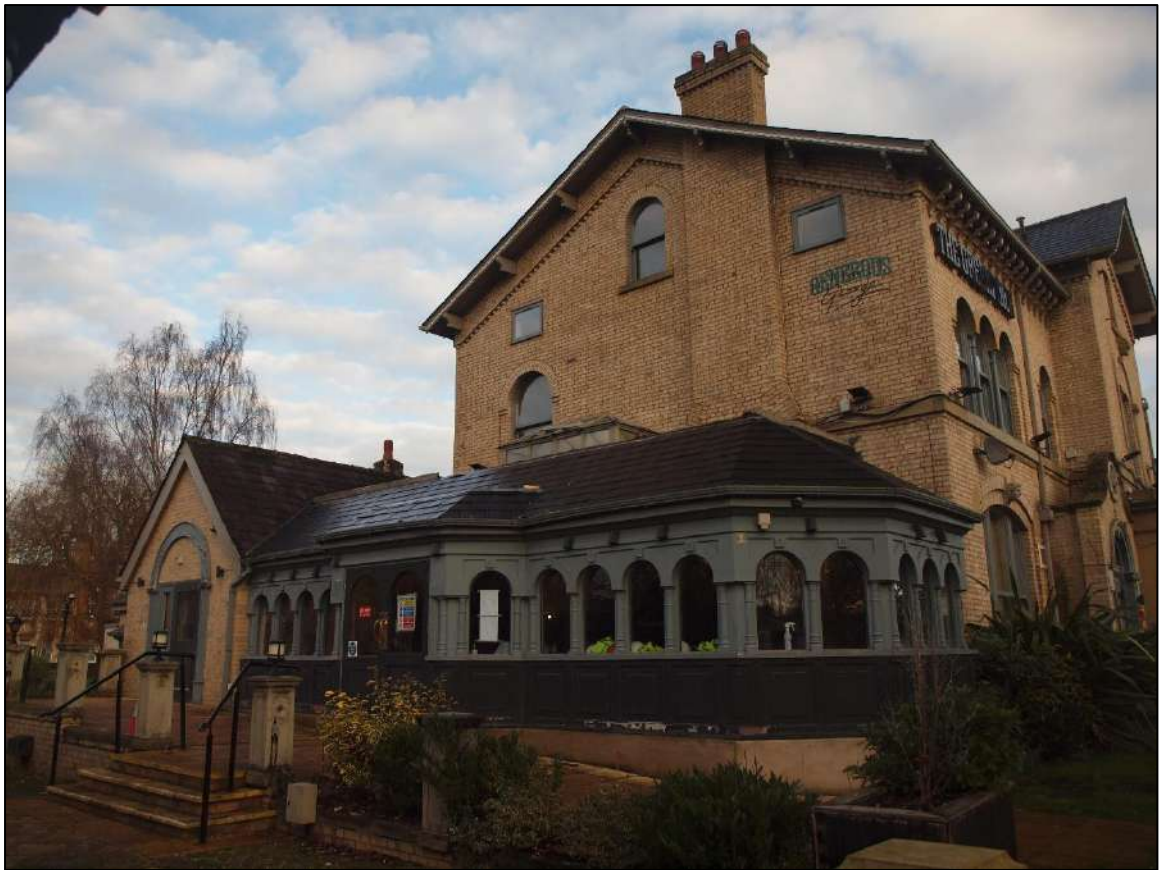
Plate 31: As above showing upper floors in gable end of house
