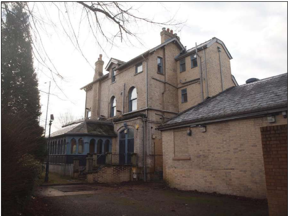
Plate 38: Northwest elevation showing stair tower
