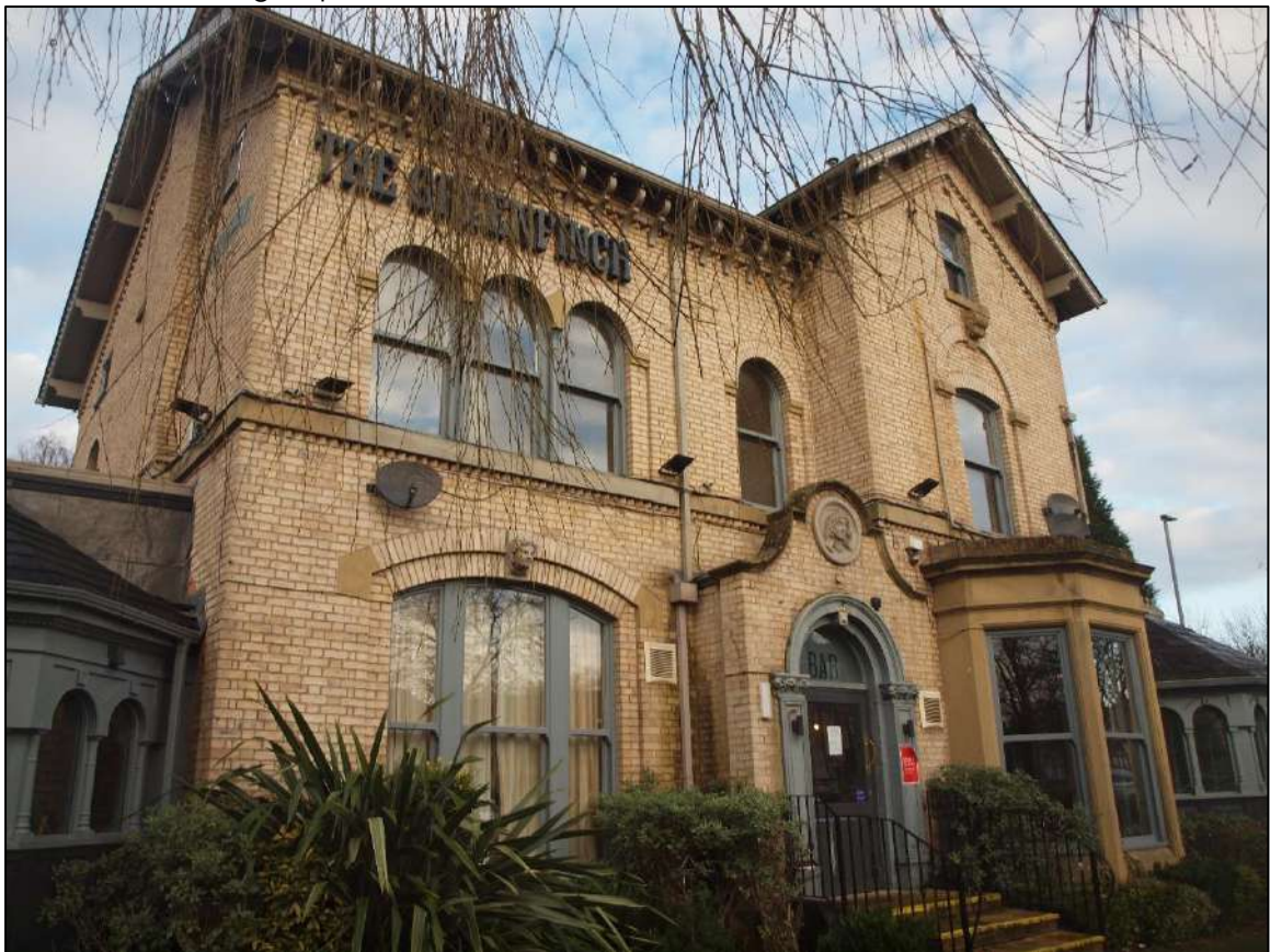
Plate 18: General shot of the southeast elevation
