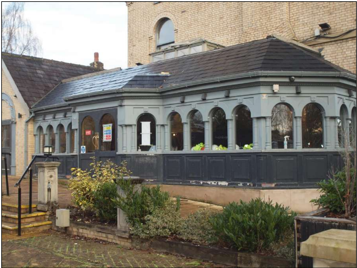
Plate 33: Modern ground floor extension
