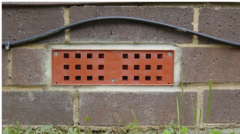
Picture 3: Example of the SMART AirBrick which has been designed to allow air to pass through freely but not water. It features simple flood activated valves that ensure compliance with BS493:1995 as an airbrick but, as soon as water enters the brick, the valves are forced closed preventing flood water from passing through.
