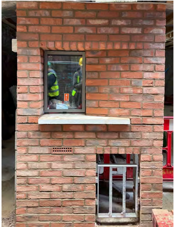
21st April 2021 inspection
