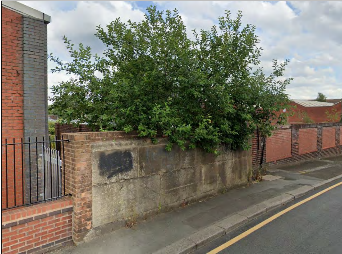
Plate 16: Canal bridge within the Site boundary at Poland Street
