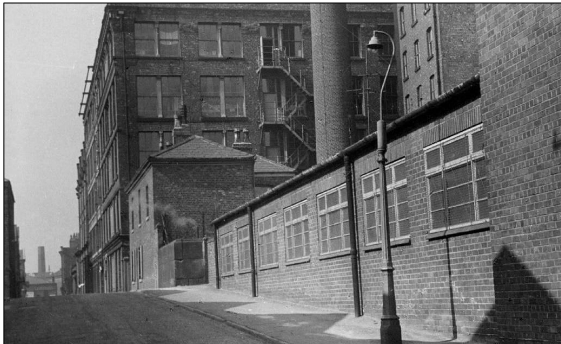
Plate 13: The clothing factory and bridge over the Bengal Arm of the Rochdale Canal on Poland Street, Ancoats, 1962
