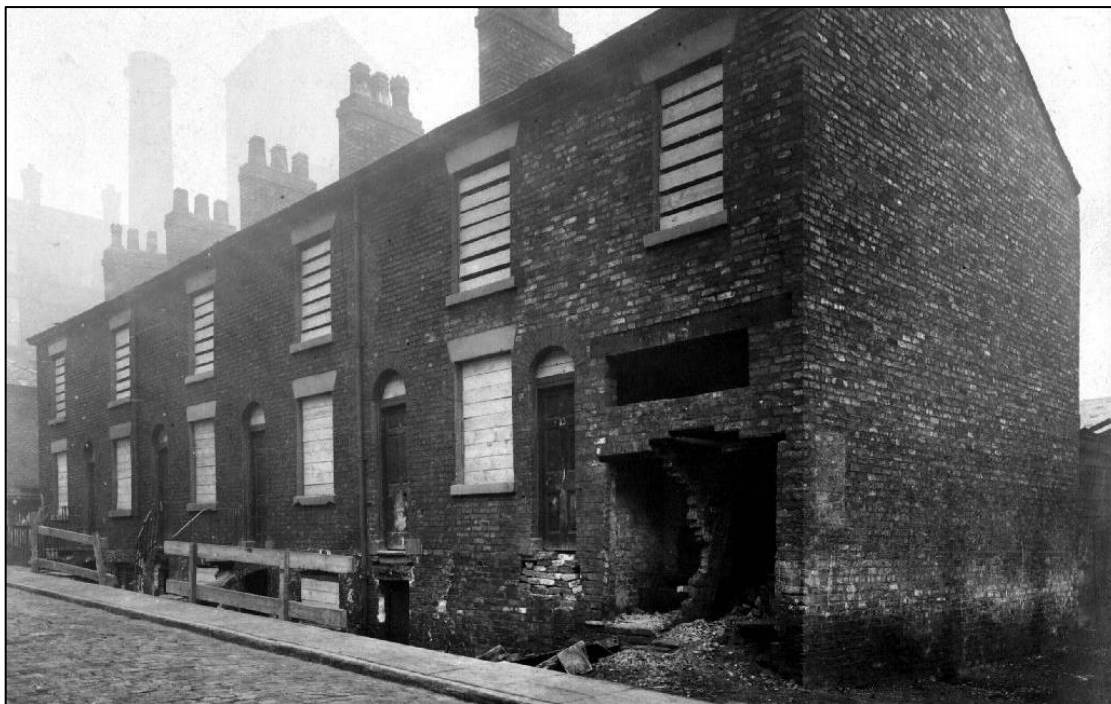
Plate 20: 55-63 Poland Street, Ancoats danger removed 7.12.1908
