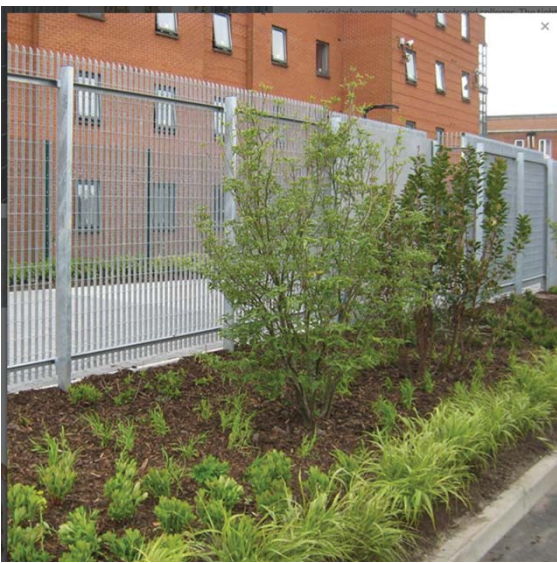
Type A steel railings
