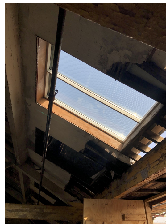
Internal images showing underside of sample refurbished roof light at No.16 Newton Street
