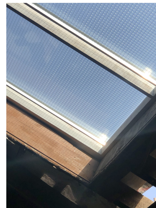
Internal images showing underside of sample refurbished roof light at No.16 Newton Street
