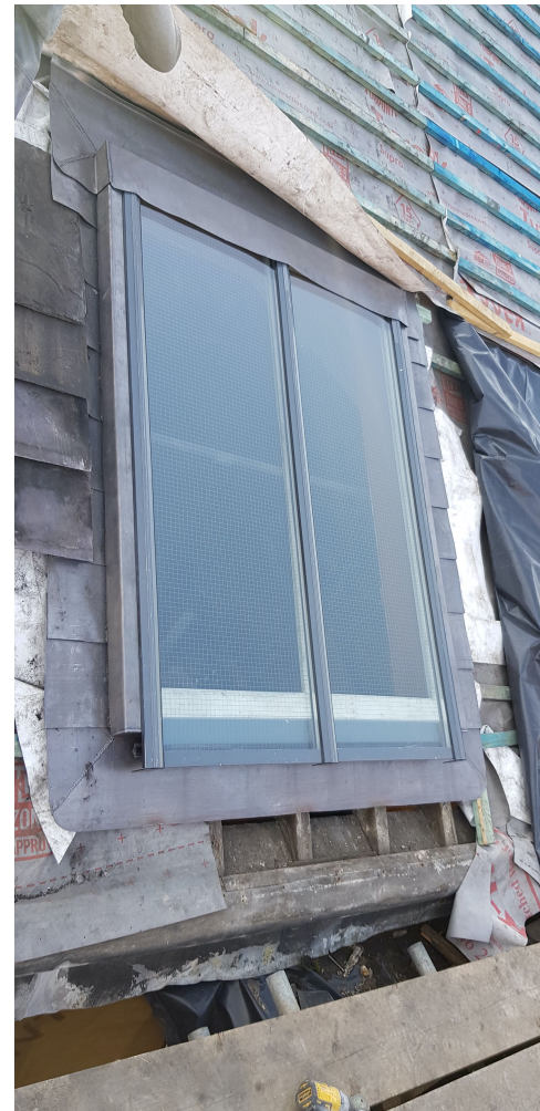
External images of sample refurbished roof light at No.16 Newton Street
