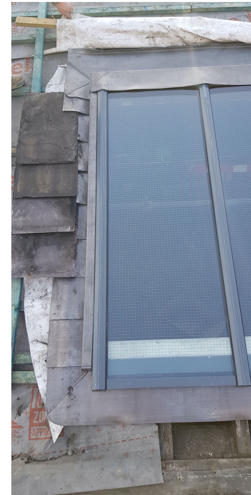
External images of sample refurbished roof light at No.16 Newton Street
