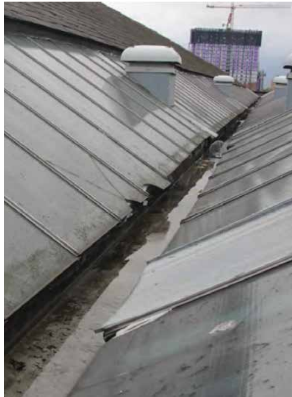
Roof gutter condition
