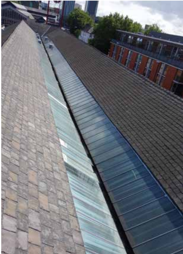
View of the slate roof and rooflights
