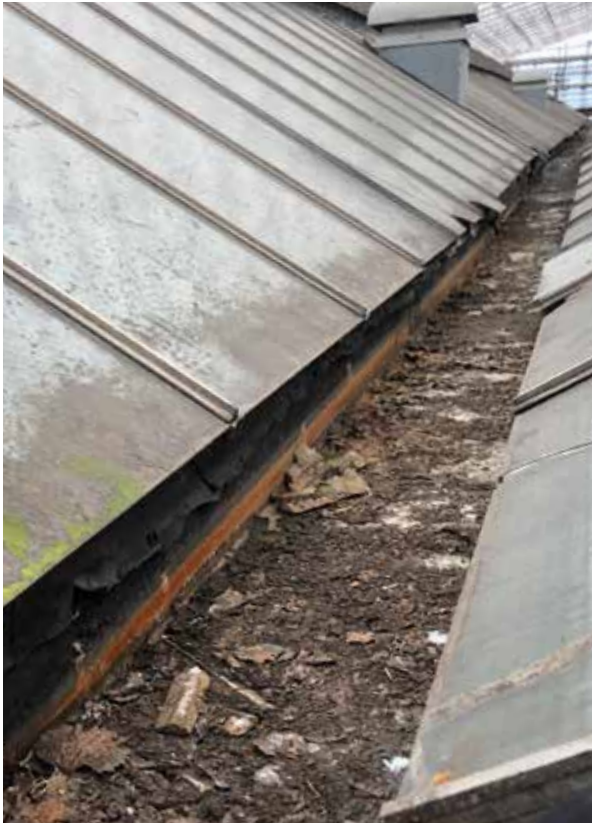
View of the central valley gutter and rooflights
