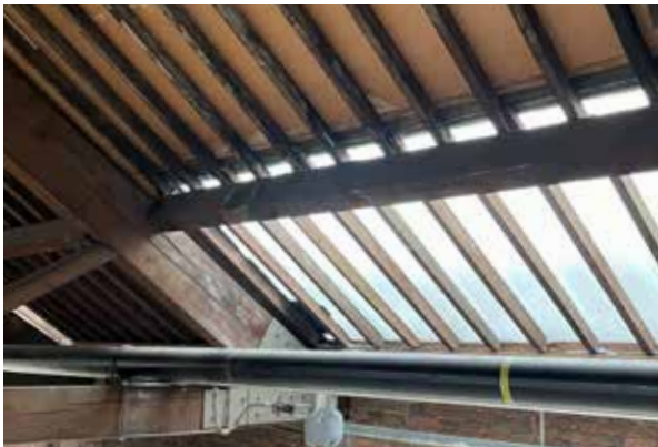
View showing modern rafters below rooflights and historic rafters above
