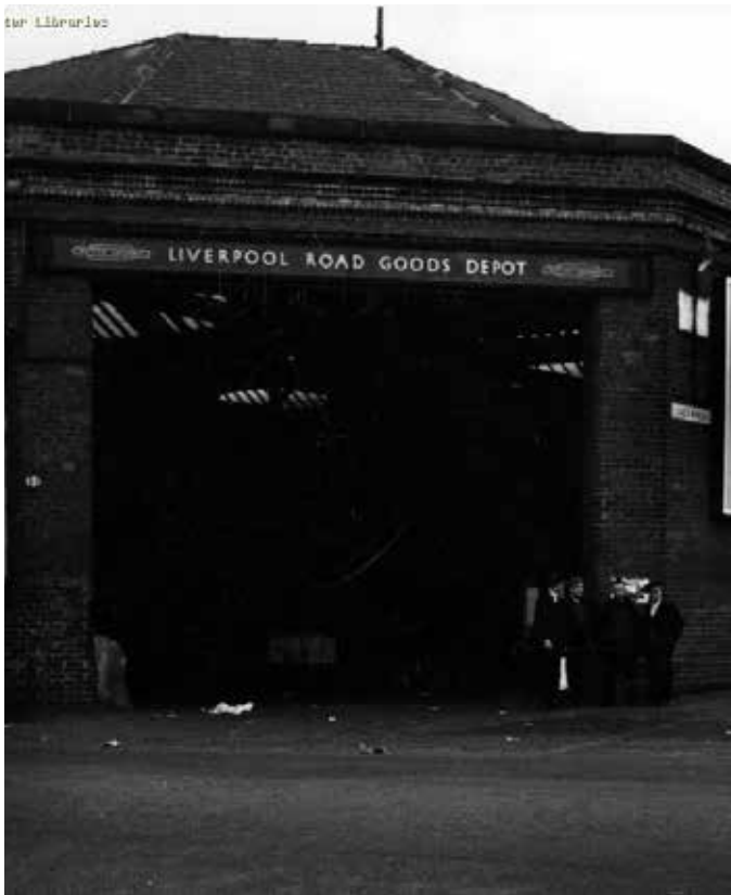
Exterior view of the Power Hall south-east, prior to restoration
