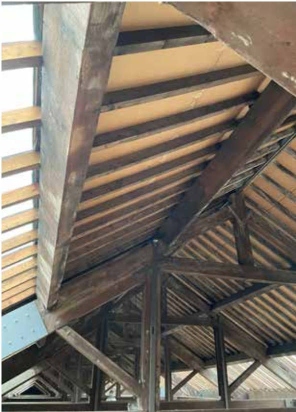
View of the existing structure and rooflights
