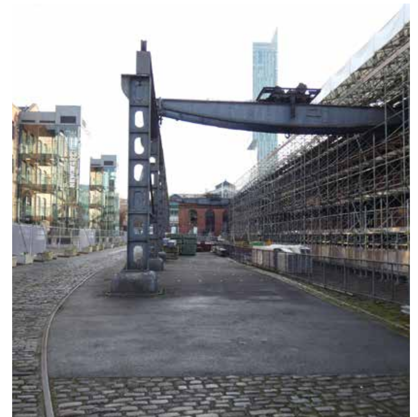
The North Yard with Power Hall (right) wrapped in scaffolding since 2019
