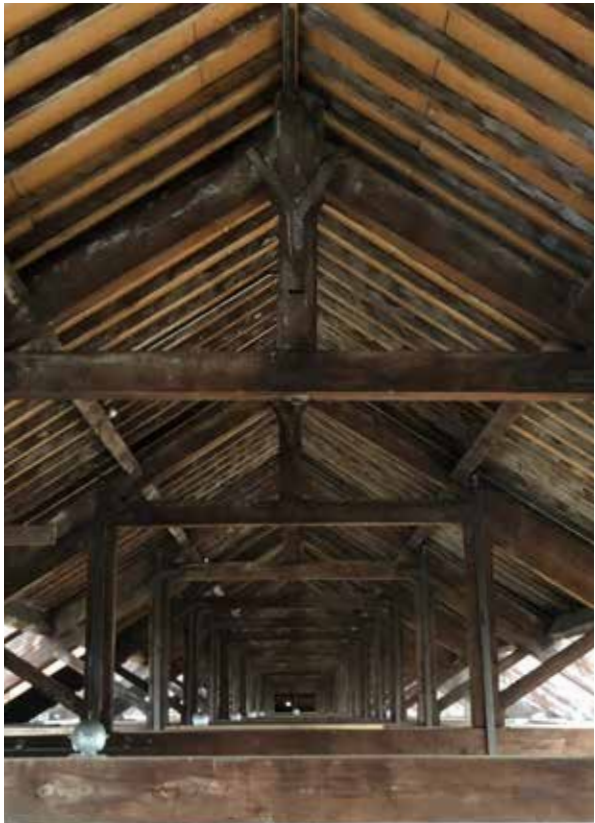
View of the existing roof structure and exposed plasterboard lining
