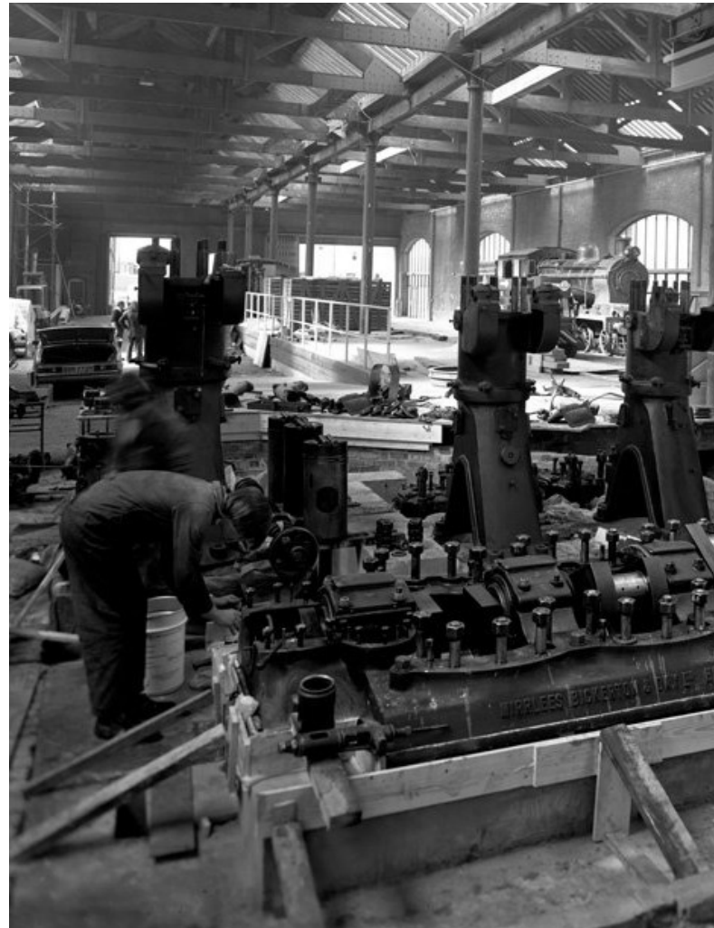
The Power Hall during 1980s restoration
