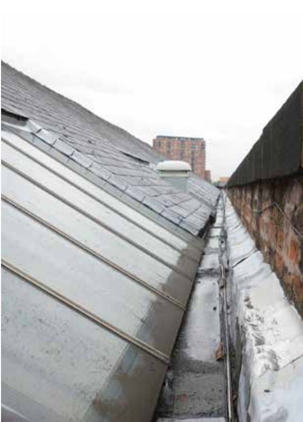
View of the parapet and outer roof pitch
