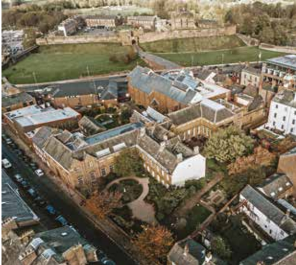
Masterplan for Grade I listed Tullie House, Carlisle.
