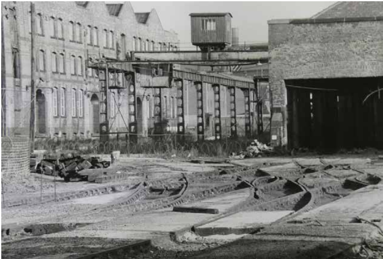
Exterior view of the Power Hall and external gantry, prior to restoration
