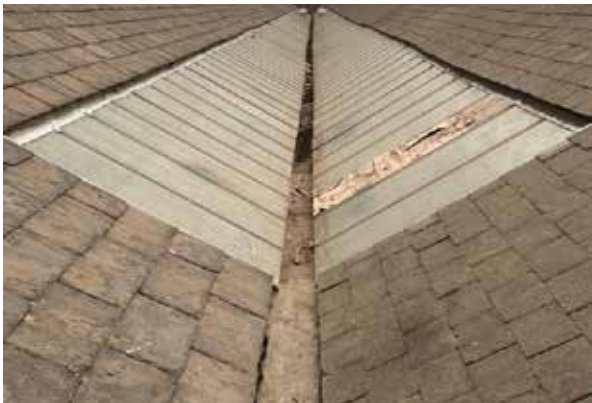
View along valley showing assumed historic slates on the left hand side
