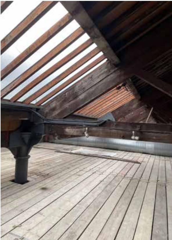
View of a typical cast iron column and fitch beam along the central valley (as seen from the temporary scaffold deck)
