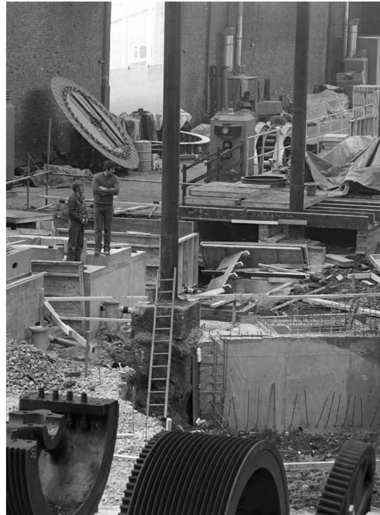
The Power Hall during 1980s restoration
