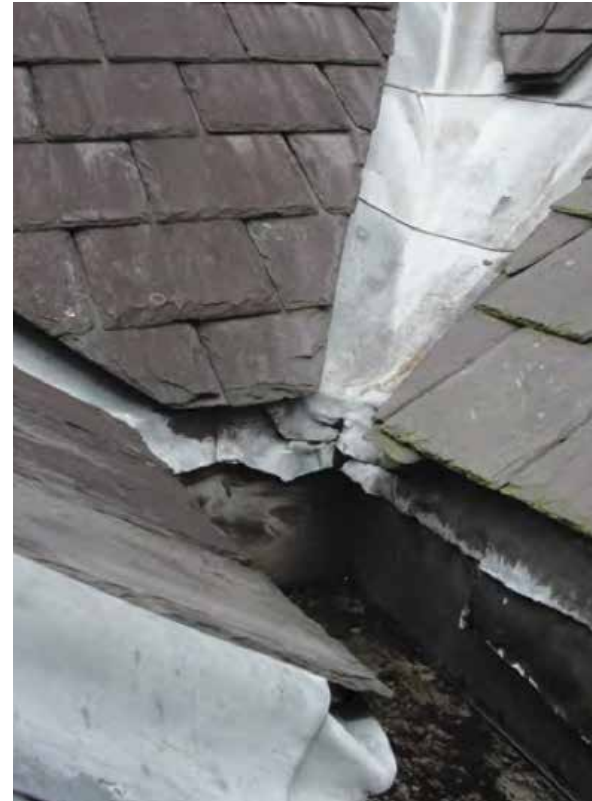
Roof gutter condition
