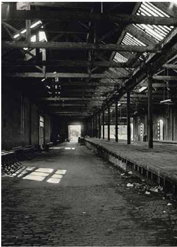
The Power Hall prior to restoration
