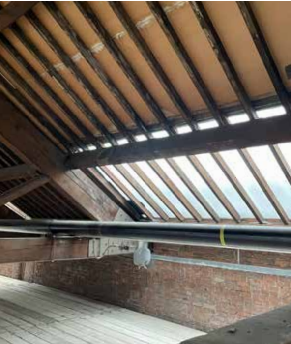
View showing modern rafters below rooflights and historic rafters above
