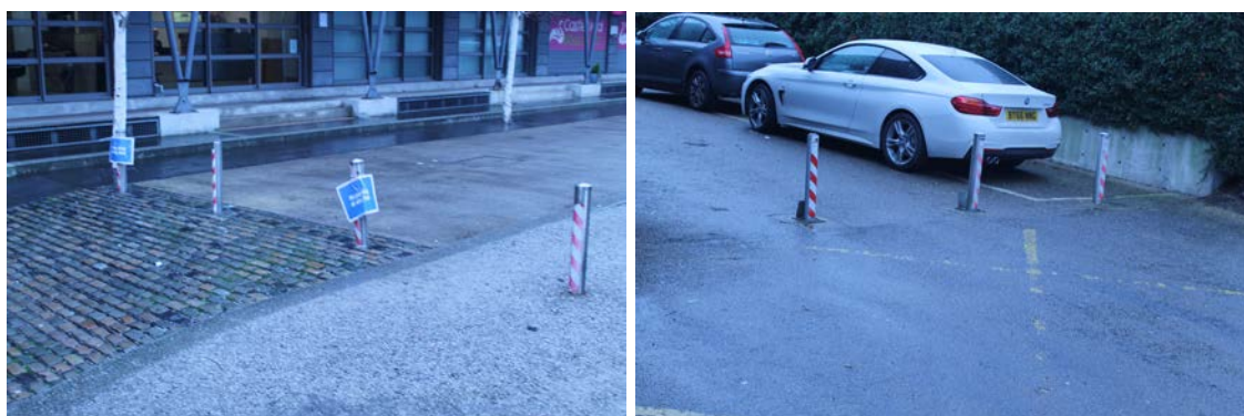
Figure A2.6 Retractable bollards blocking access to the rear of Gym and urban splash building
