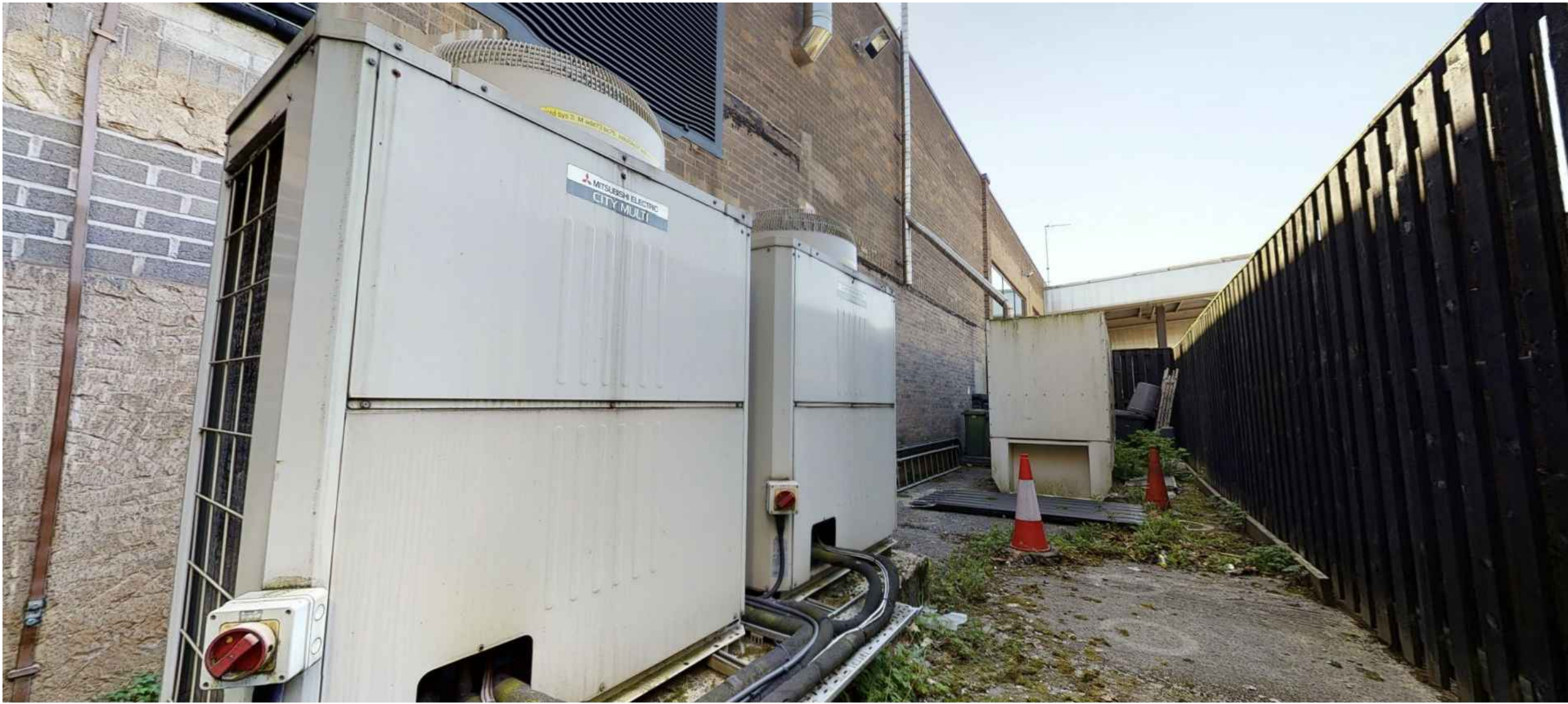
Existing External Compound
